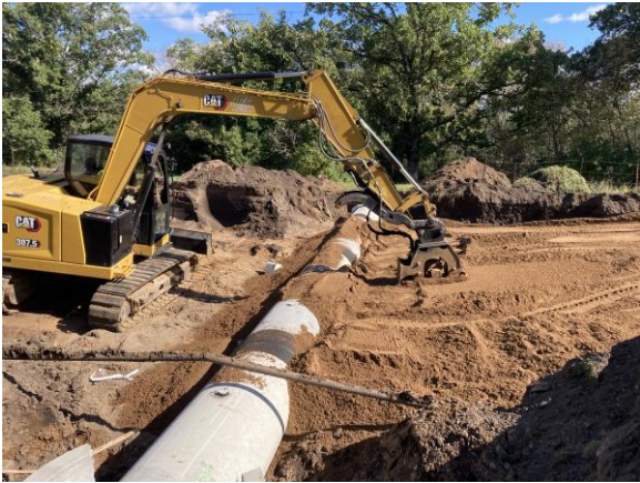
(c) Compaction of backfill
