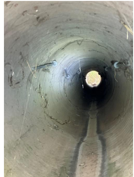
(b) Culvert 2183548 in District 2, Interior Ties
