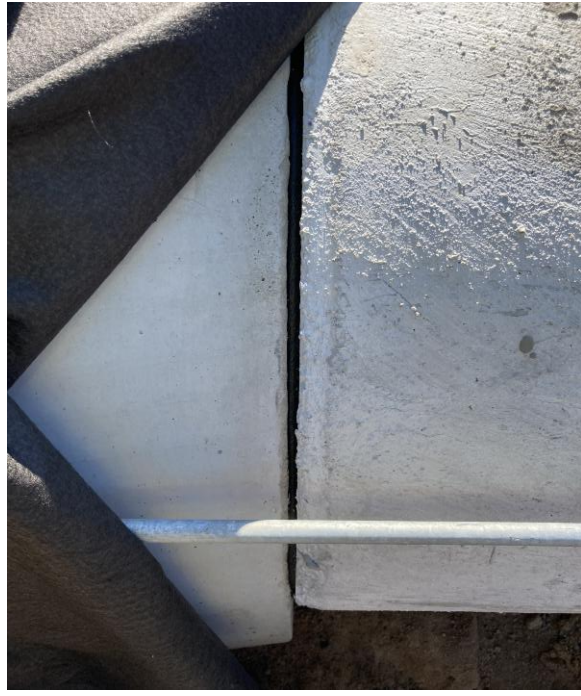
(b) Typical joint with mastic seal
