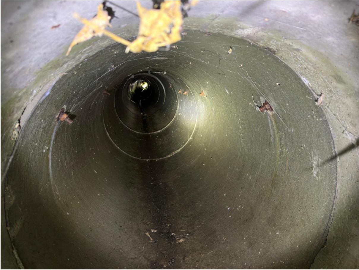
Figure 1 - a culvert in district 8 with pipe ties just to third segment
