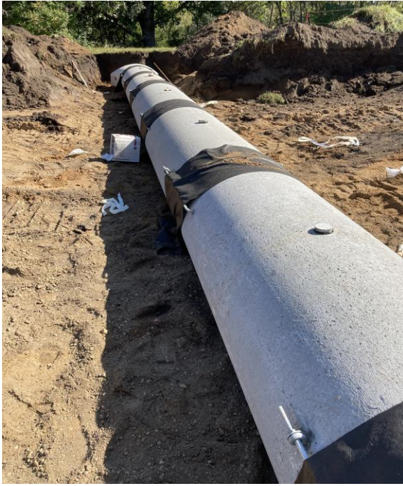
(a) Pipe prior to backfill
