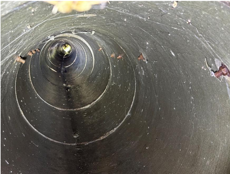
(a) Culvert 2207834 in District 8, Exterior Ties
