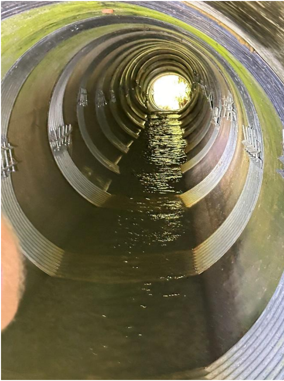
(c) Culvert 2214249, District 7: Metal bands
