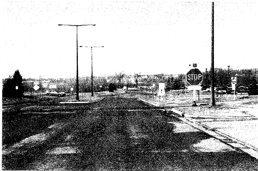
Figure 3. View of the STOP sign and red warning light at Westgate and Transitway.
