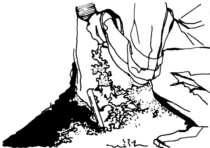
Figure 4: Weep-pipe installation
