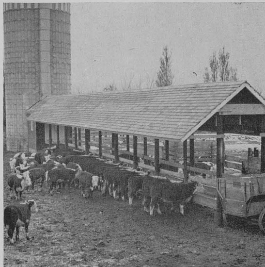
A shed with an overhead track reduces labor of handling silage. Note feed wagon at end of track for convenience in feeding.
