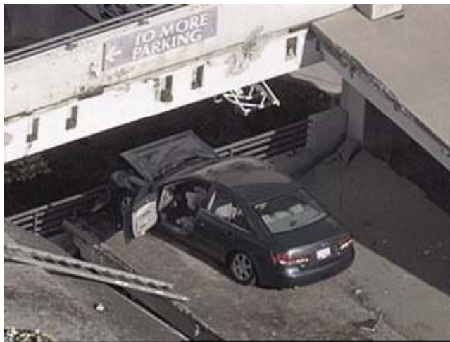
(b) Close-up of the failure
