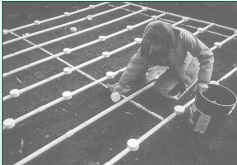
NRRI researcher Barb McCarthy installs pieces of the distribution network on an in-ground peat filter at the test site near Duluth.
