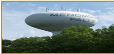
Pictured: Menomonee Falls Water Tower
