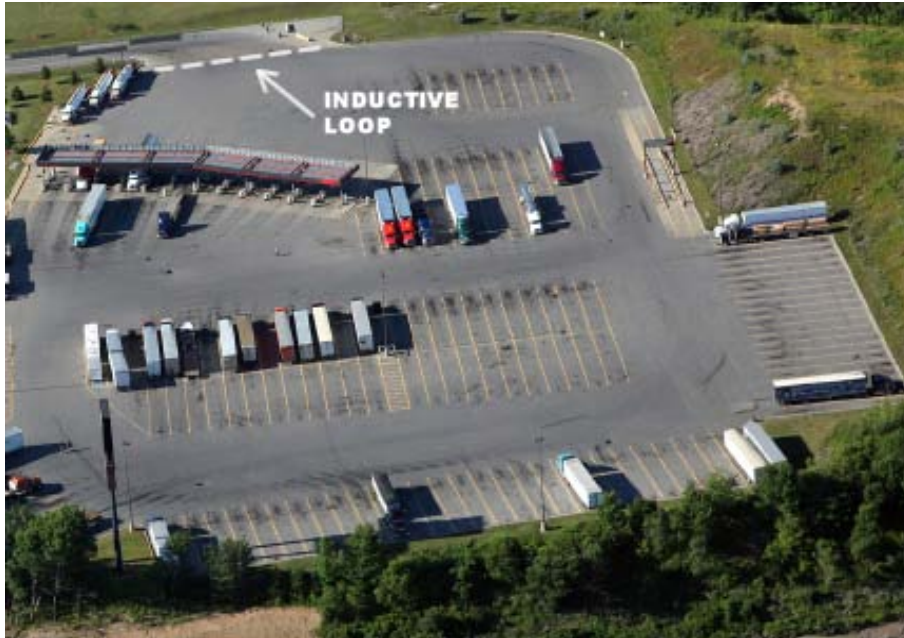
Figure 3 – An illustration of a truck stop with an inductive loop at the entry/exit.
