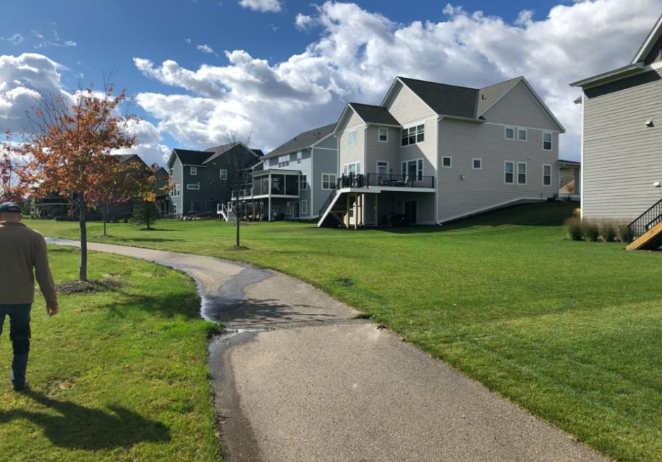
Water pooling on the walking trail
