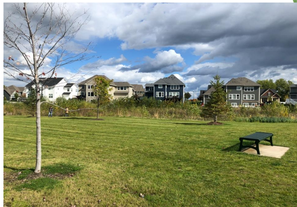
Standing water near the retention pond
