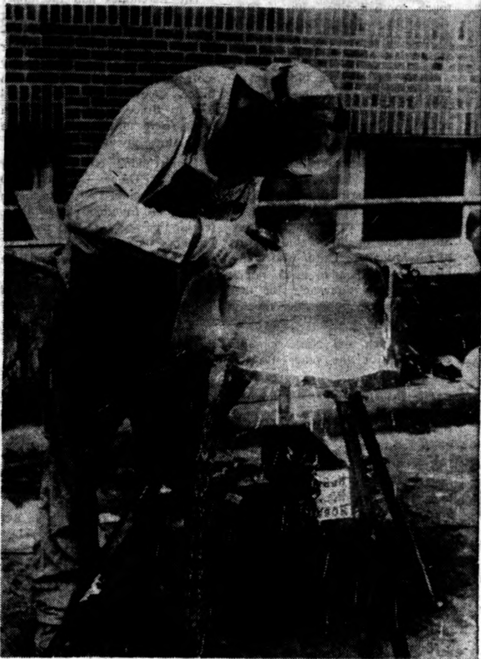
The use of steel requires techniques foreign to many people. This worker is operating an arc welder, which is used to join pieces of steel.
