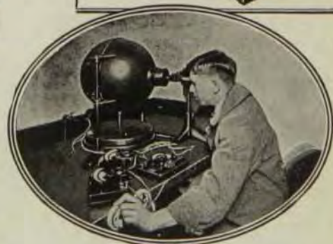
Looks like a bomb, but really a little "dark room" which permits the inspector to know exactly whether a tiny switchboard lamp comes up to the mark.
