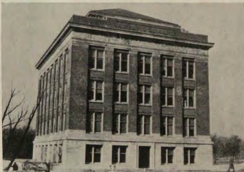
A View of the New $250,000 Botany Building
