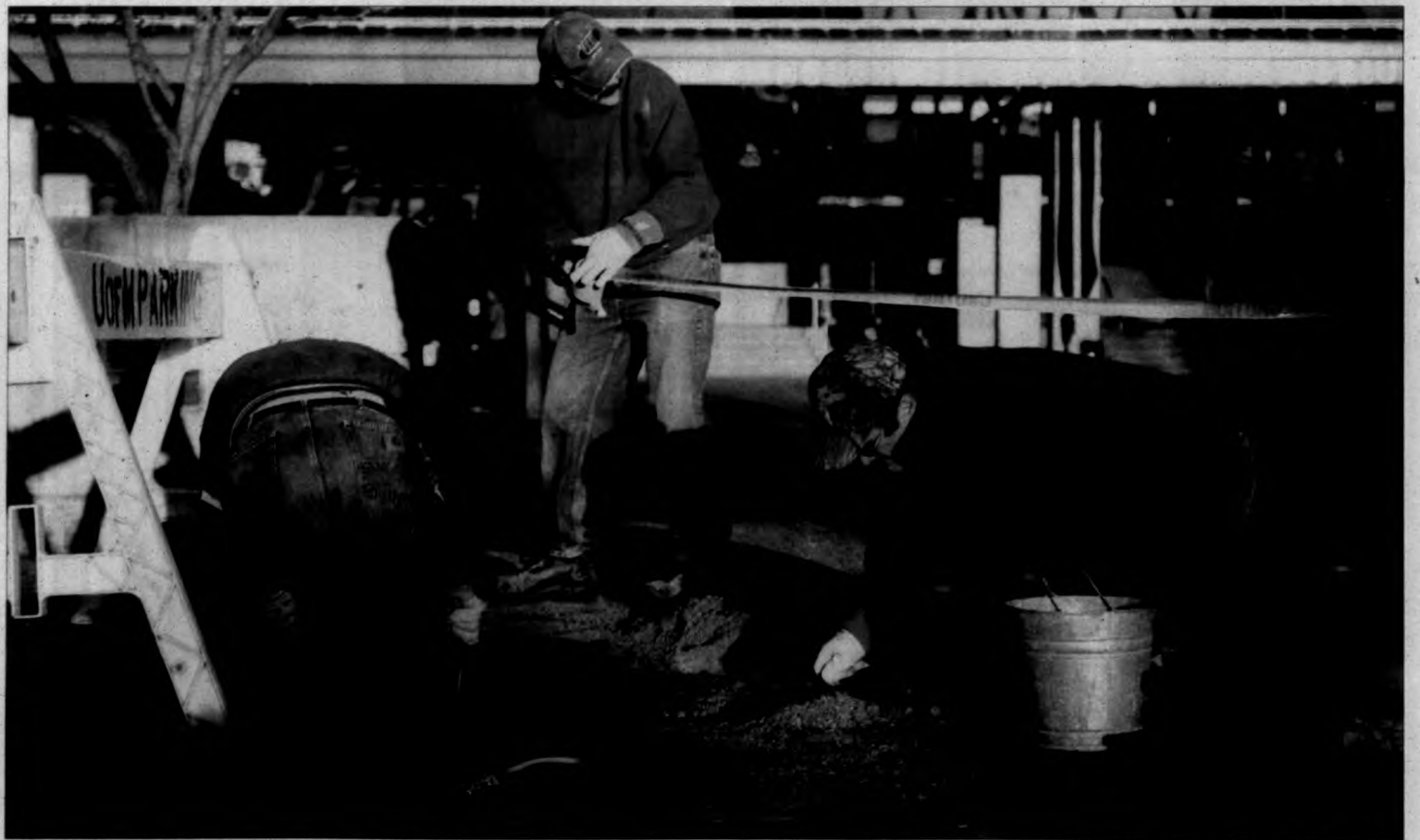
7:01 a.m. Facilities Management workers Craig Dircks, left, Dale Carlson and John Kohman repair stone tiles on David Lily Plaza on the east side of Northrop Auditorium. ERIC SWANSON
