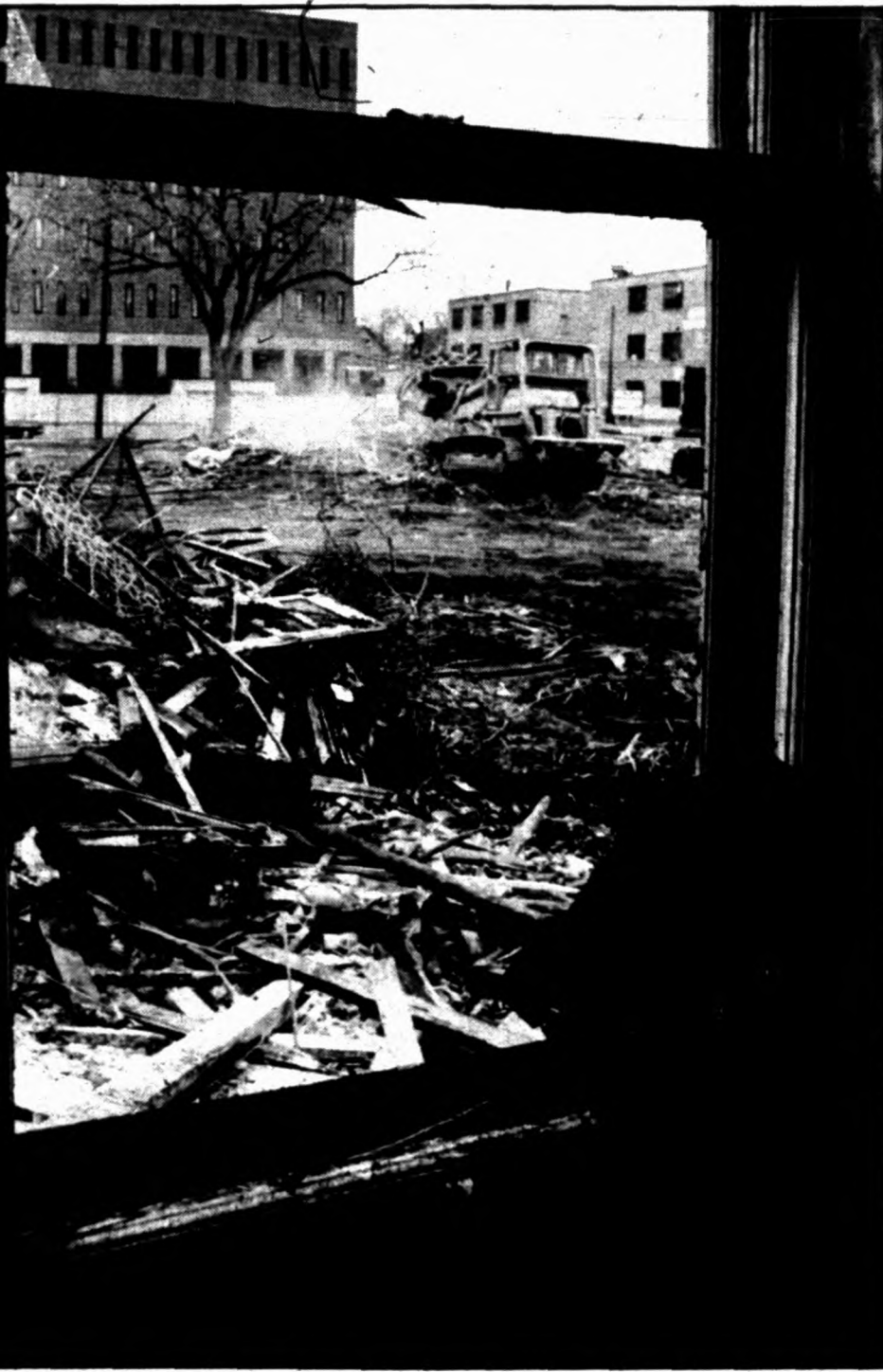
BULLDOZER CLEARS THE WAY
