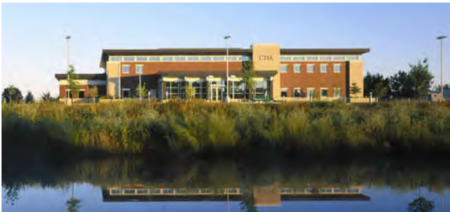
Dakota County CDA building, www.dakotacda.org
