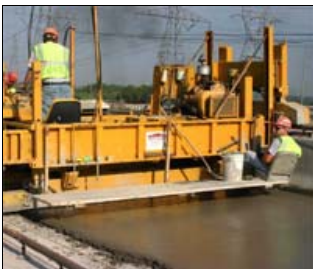
Workers replace a concrete bridge deck
