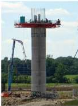
Figure 2.10. Jump forms used in concrete tower construction [7].
