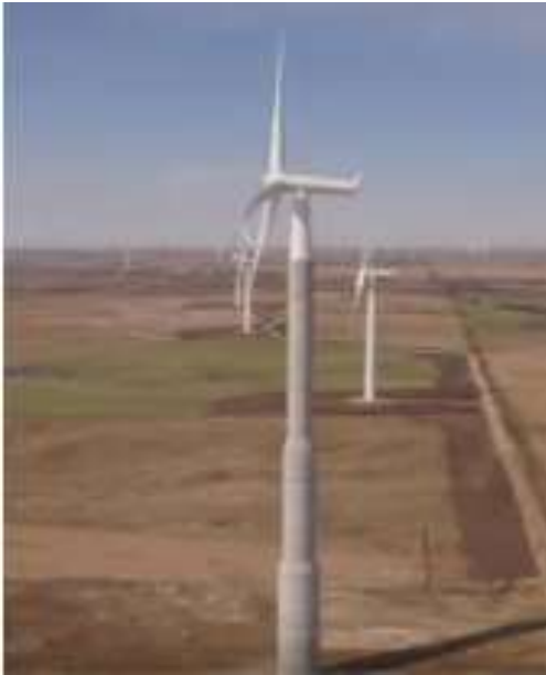
Figure 2.7. MidAmerican hybrid tower [28].
