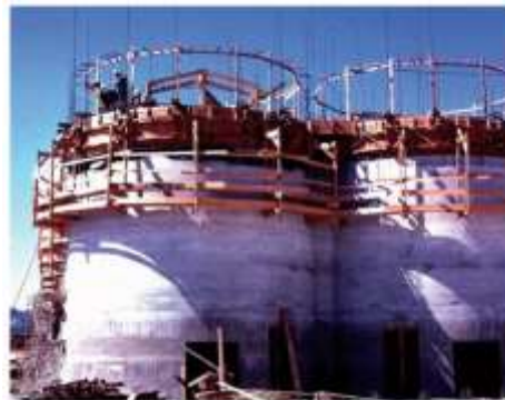
Figure 2.11. Slip forms used in grain silo construction [7].
