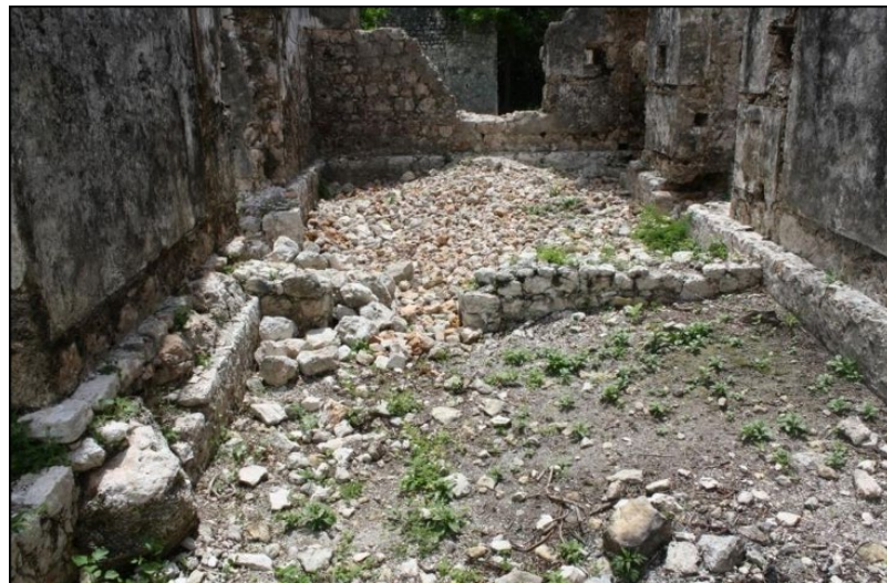
Figure 5.11: Space 105 looking west from Space 106 (JNHT 2010: 15)
