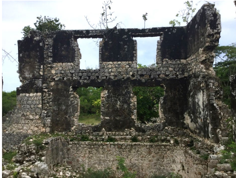
Figure 5.7: Western wall of spaces 001, 101, and 201.
