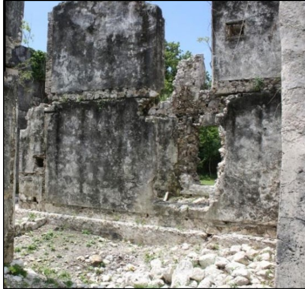
Figure 5.10: Space106/206 looking north from Space 103 (JNHT 2010: 15)
