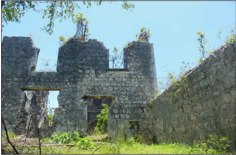
Figure 5.13: Exterior image of east wall of spaces 103 and 203, highlighting the disjunction of alignments of doors and windows.
