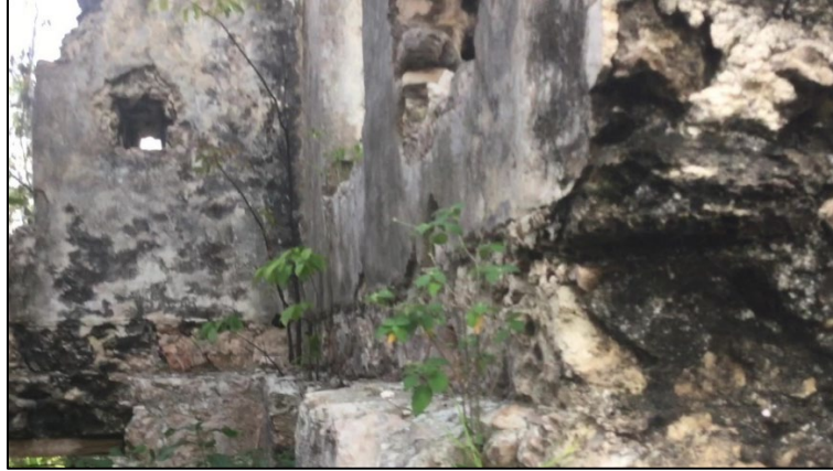
Figure 5.21: Interior western face of south tower, demonstrating continuity of baseboard and sill between tower and space 102.
