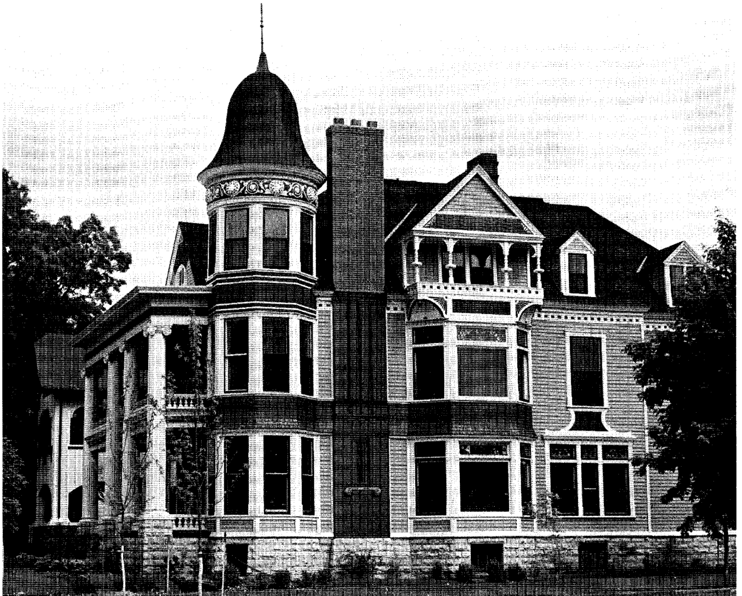
The Historic Hill Area in St. Paul combines condominium conversions with rehabilitations.
