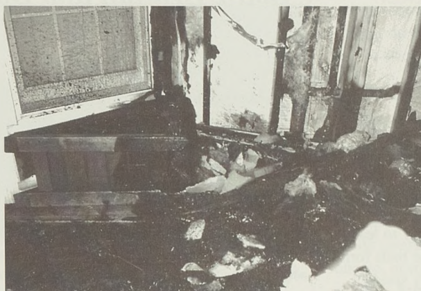
Spontaneous combustion nearly led to disaster. A planter identical to the one at far left was filled, prior to planting, with peat, nitrogen pellets, and fertilizer. The planters both had drainage holes in the bottom. They sat all summer on a deck that faced south. Fire officials ruled out several possible causes—e.g. dryer vent, cigarettes—and deduced that the planter overheated as the sun's path shifted and light shone more directly onto the planter in early September, when the fire occurred. Photos courtesy Chanhassen Fire Department
