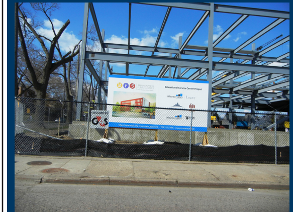
Minneapolis Public Schools' Educational Service Center Project
