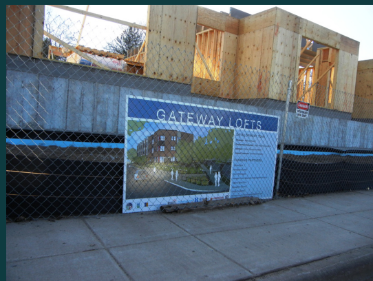
Gateway Lofts Development
