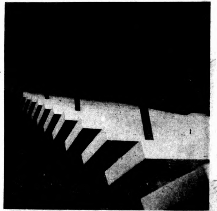
The steps leading to the second floor are cut from solid stone. The building was first planned in 1944
