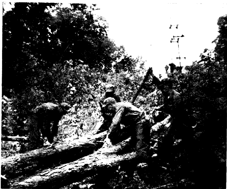
Minnesota cadets cutting timber piles for bridging.
