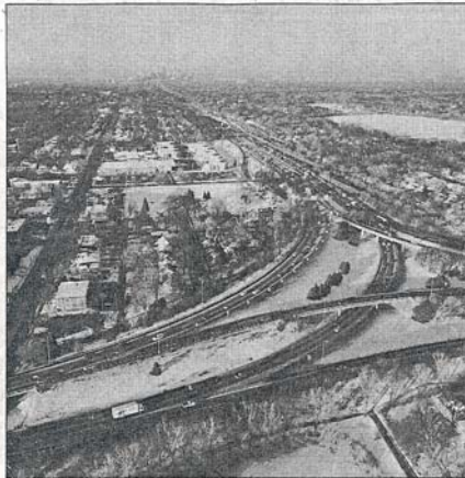
Star Tribune photo by David Brewster The Interstate Hwy. 35 and Crosstown Hwy. 62 bottleneck. "Congestion pricing" could manage traffic and bring in revenue without toll booths.
