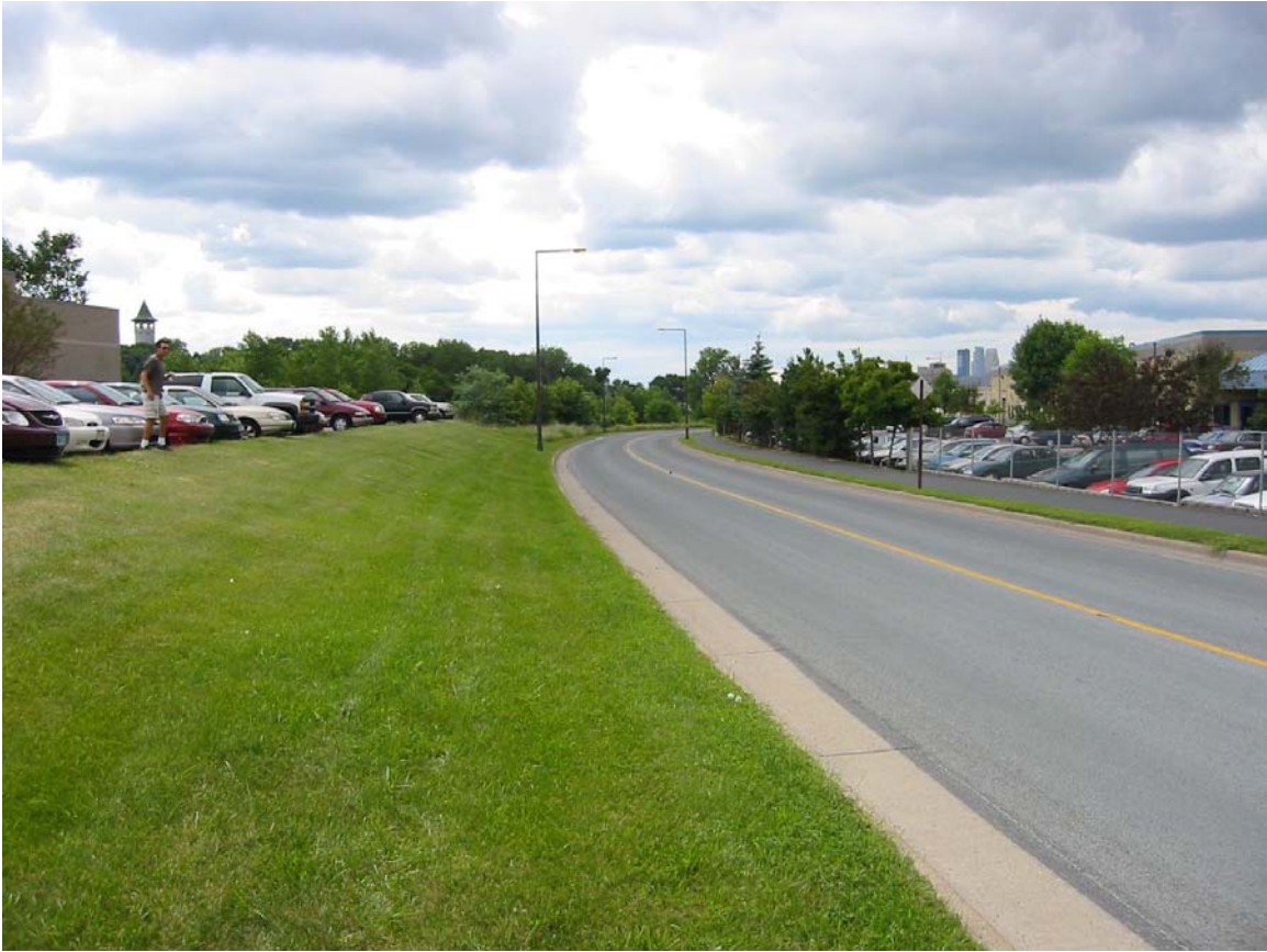
Picture 5. Photo of Transitway looking west at the Westgate intersection.
