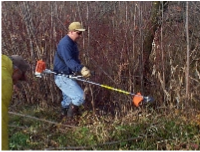
Figure 6.10 Power trimmer used to cut plant materials for fascines and brush mattress.
