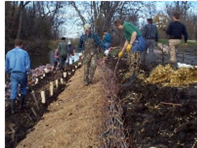
Figure 6.13 Installation of horizontal fascines; coir mesh, seed & mulch between fascines.
