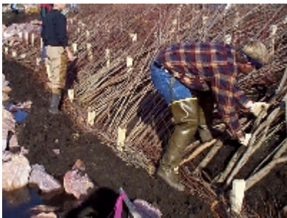
Figure 6.18 Placing cuttings in brush mattress.
