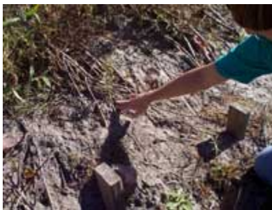
Figure 6.29 Growth coming where willow ends covered with soil.
