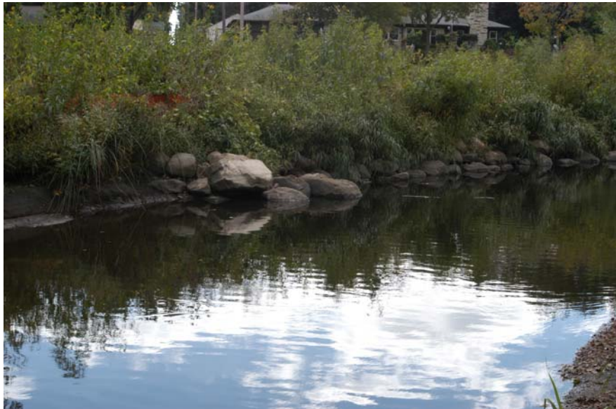
Figure 6.8 Rock vane, boulder toe, and willows.
