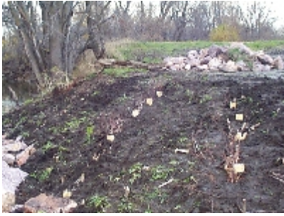
Figure 6.16 Diagonal fascines to convey water and take up water along slope.
