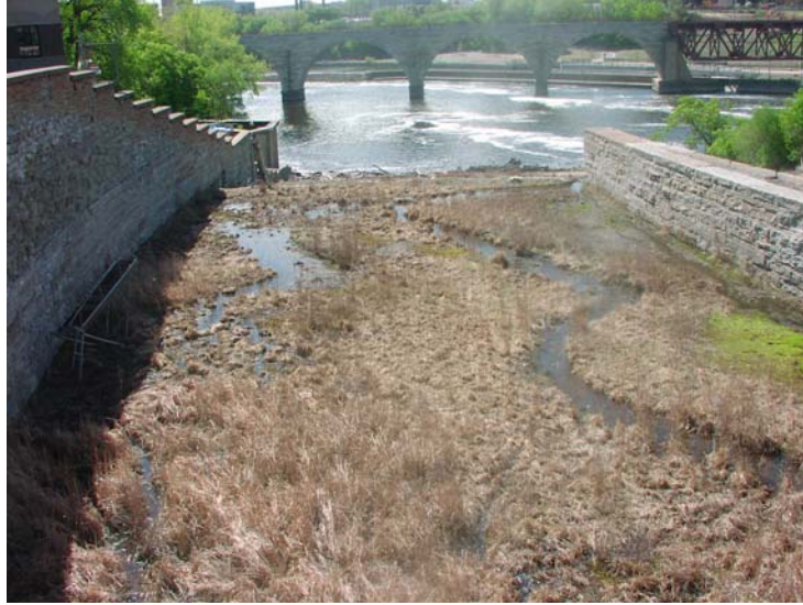
Figure 8.15 Wasteway no. 2: View from upstream looking downstream.
