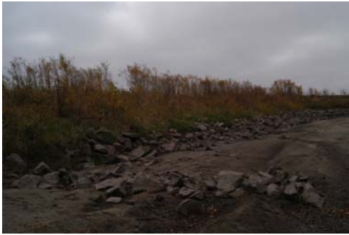
Figure 6.30 Looking upstream. Fascines are in the foreground and brush mattresses are in the background.
