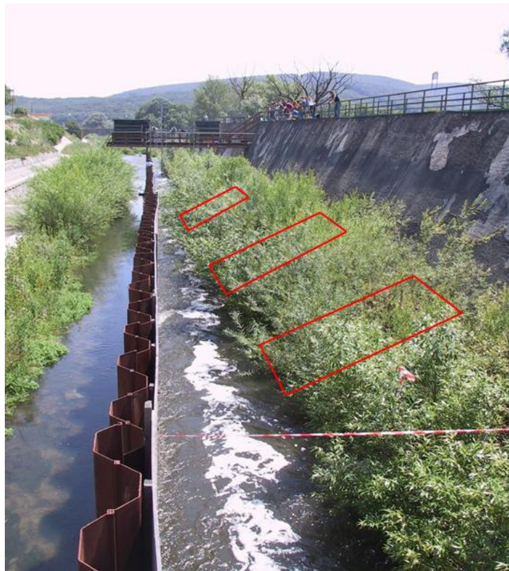
Figure 8.7 View from upstream to downstream of the flume.
