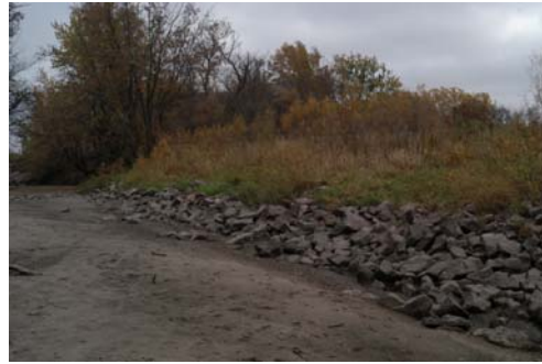
Figure 6.31 Fascine area, looking downstream.
