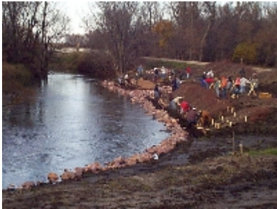
Figure 6.12 Fascine installation on northern end of site; brush mattress on southern end; rock toe to channel forming discharge.
