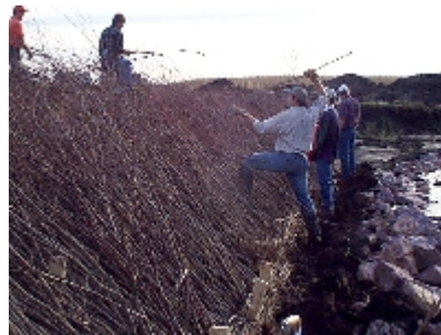
Figure 6.19 Brush mattress constructions.
