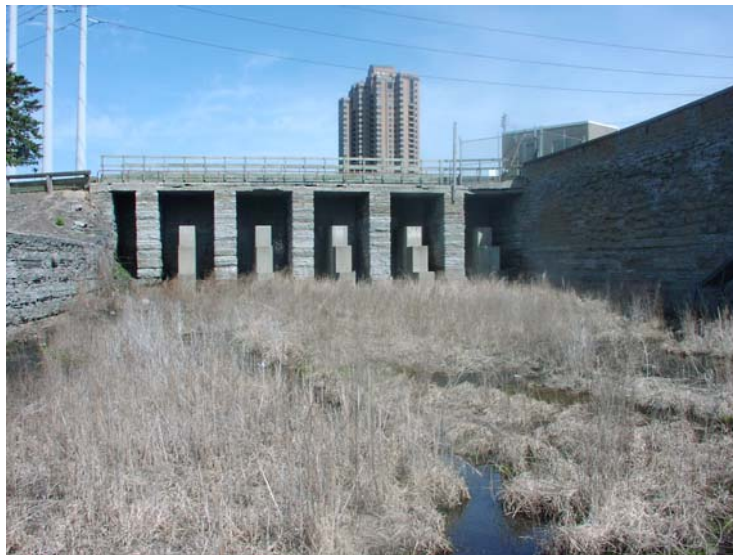
Figure 8.16 Wasteway no. 2: View from downstream looking upstream.
