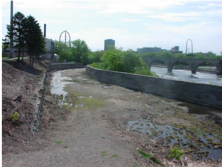
Figure 8.13 Wasteway no. 1: View from upstream looking downstream.
