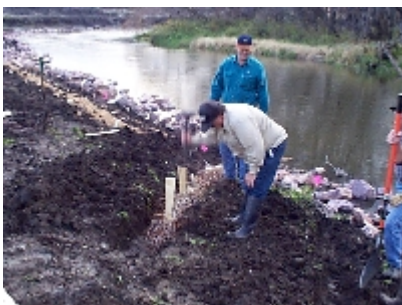
Figure 6.14 Installing diagonal fascines.
