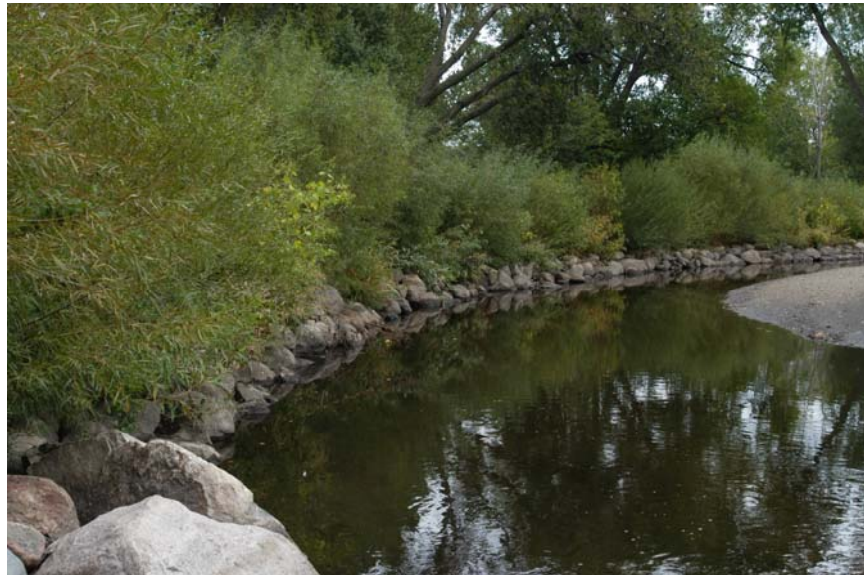
Figure 6.6 MHC site at 18 th Ave. S. Boulder cover below, willows on top of bank.
