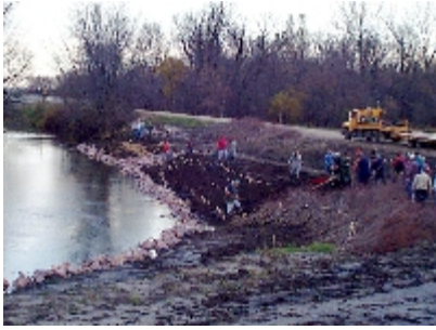
Figure 6.22 Project nearing completion; fascines on north end and brush mattress in foreground.
