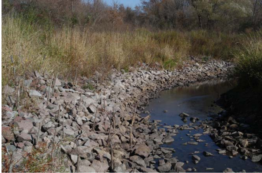
Figure 6.4 Dead willow posts in the riprap.
