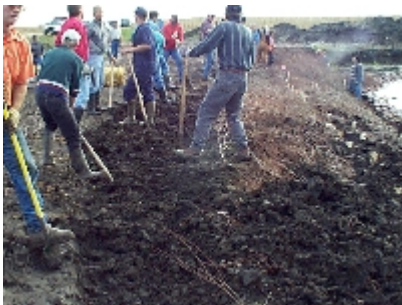
Figure 6.20 Covering brush mattress with topsoil (soil was to wet for machinery).
