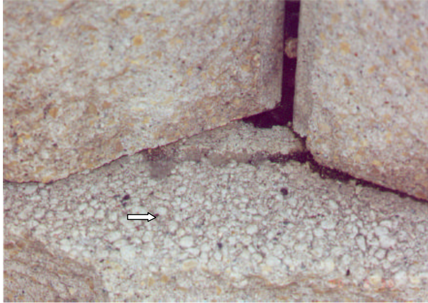
Medium-Severity Erosion
