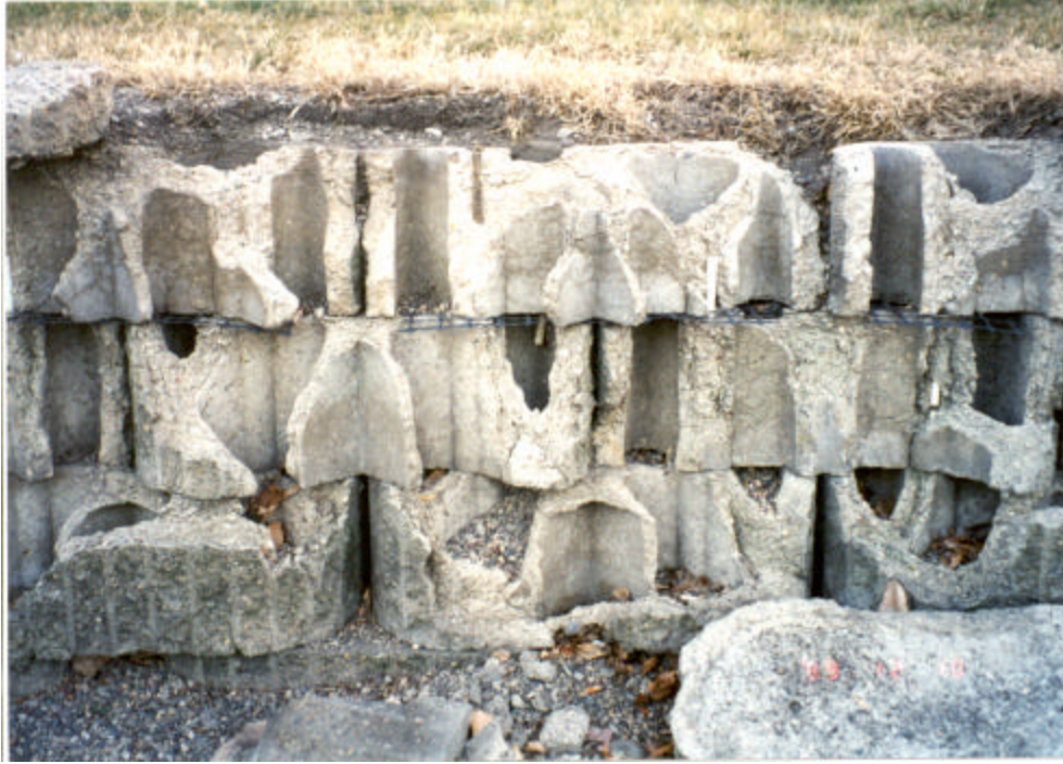
Figure 4.11. Close-up photo of high-severity scaling on SCBRW subjectively rated as “very poor”.
