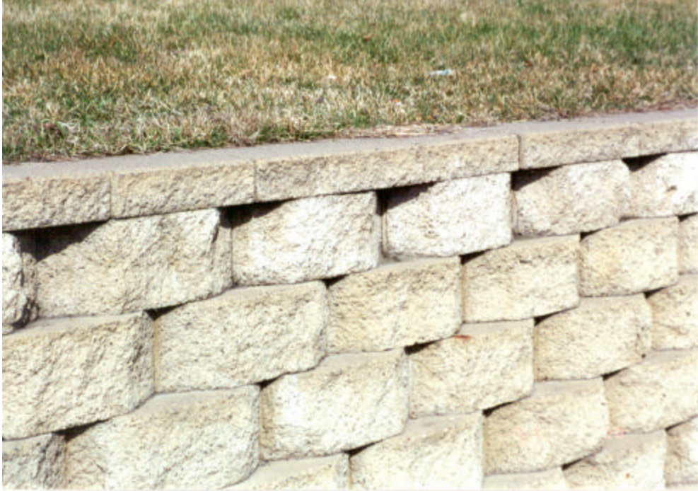
Figure 4.27. Photo of general condition and low-severity freeze-thaw damage of masonry units used in SCBRW subjectively rated as “good”.
