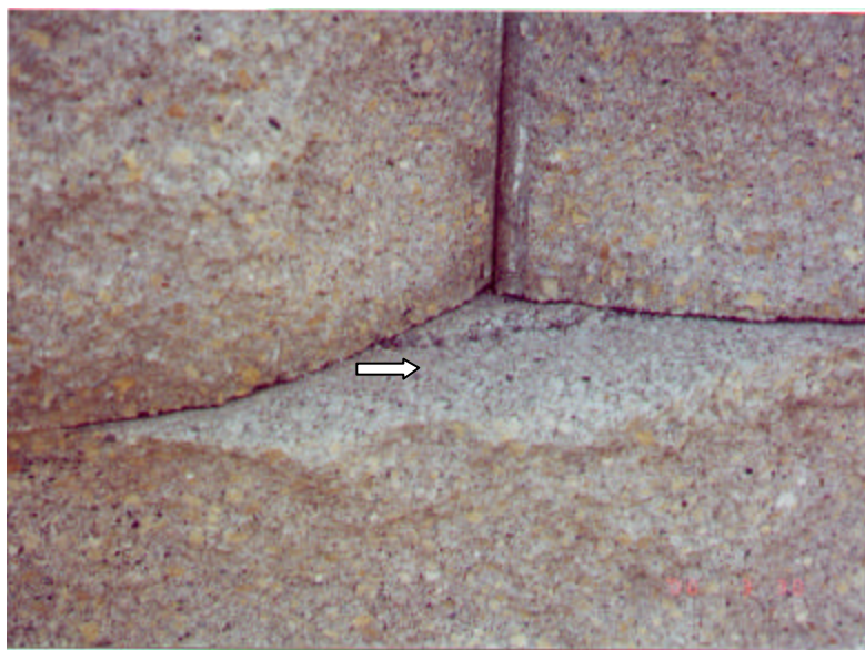
Low-Severity Erosion
