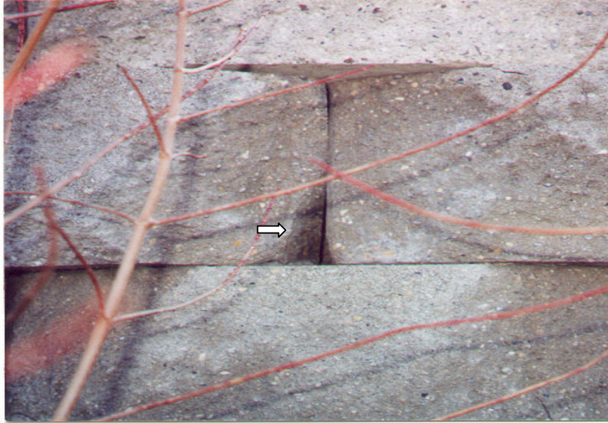
Medium-Severity Spalling
