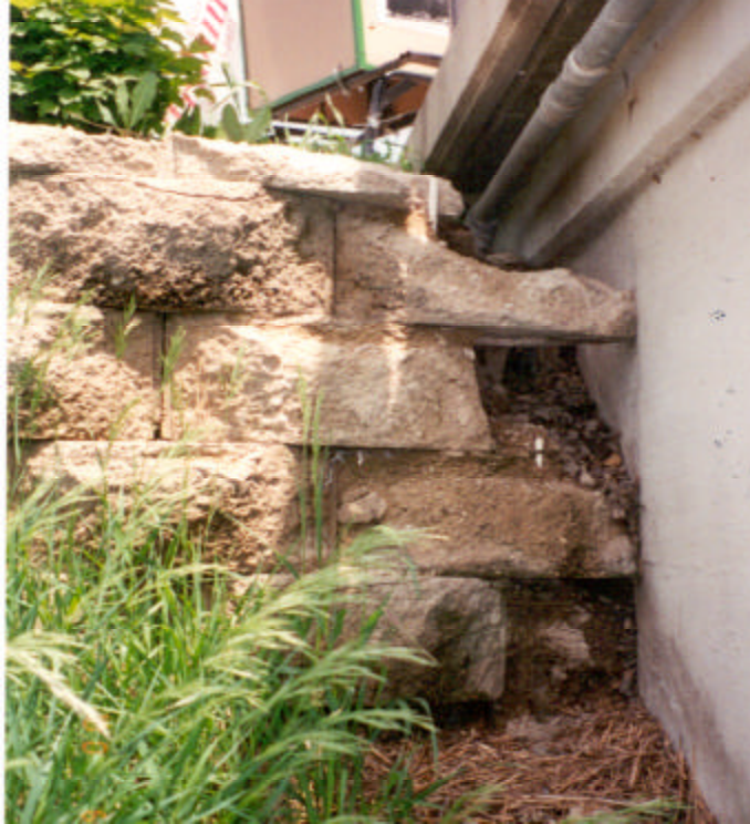
a. SCBRW located on west side of pedestrian bridge.
