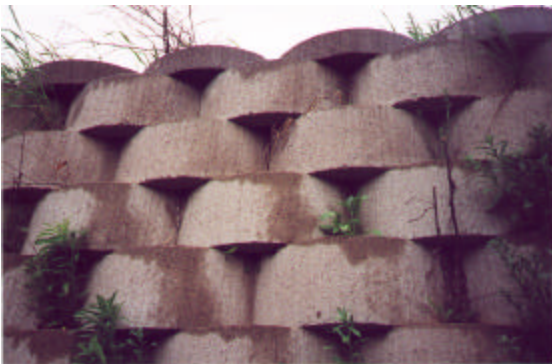
Low-Severity Embedded Vegetative Growth
