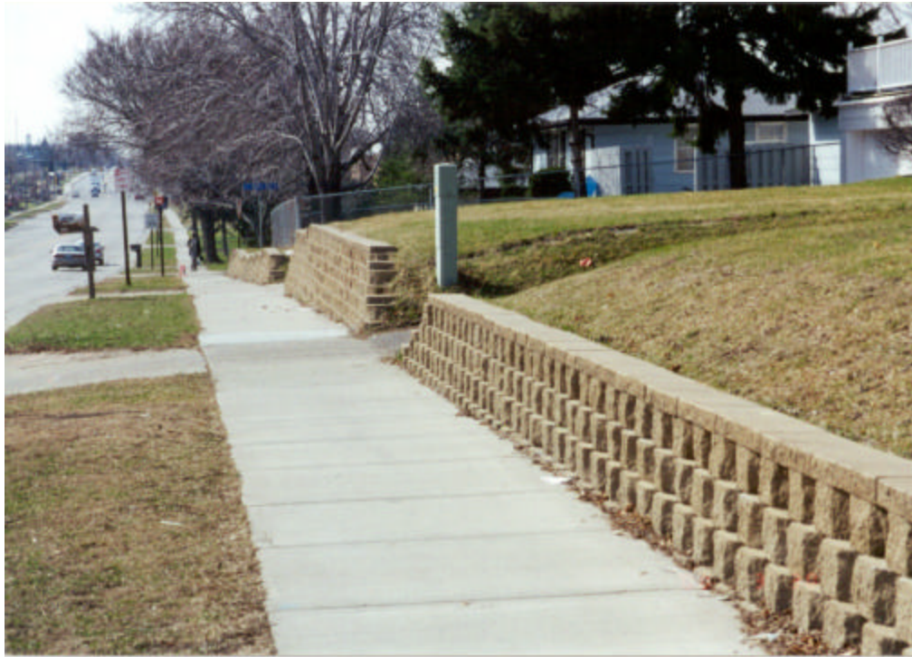
Figure 4.25. Overall condition photo of SCBRWs subjectively rated as “good”.
