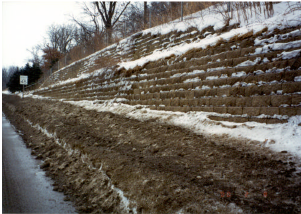
Figure 4.17. Photo illustrating high quantity of deicing sand/salt in snow accumulation.
