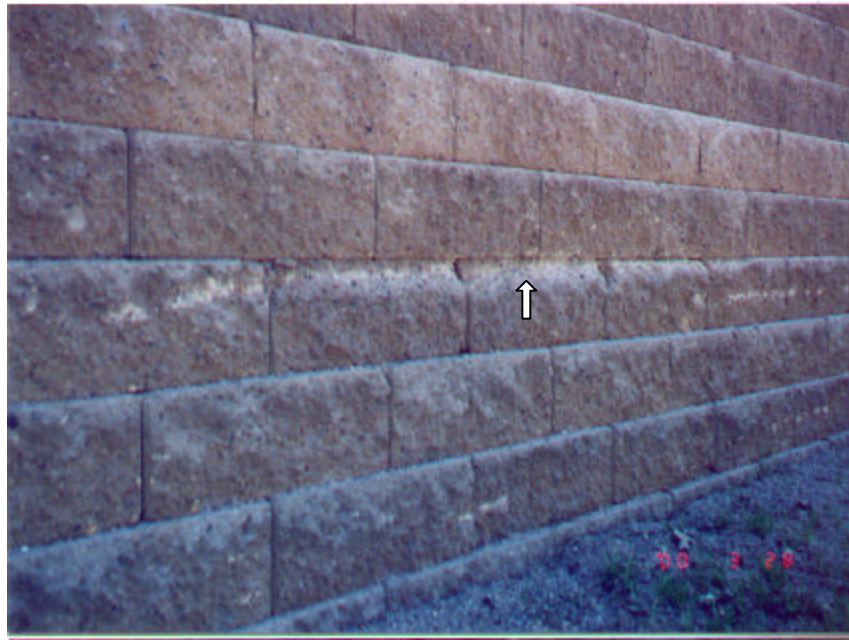
Scrapes in Vertical Surface Block
