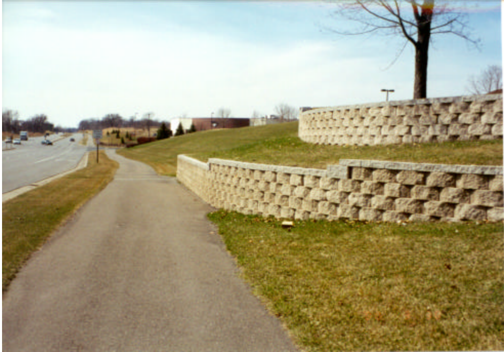
Figure 4.31. Overall condition photo of SCBRW subjectively rated as “very good”.
