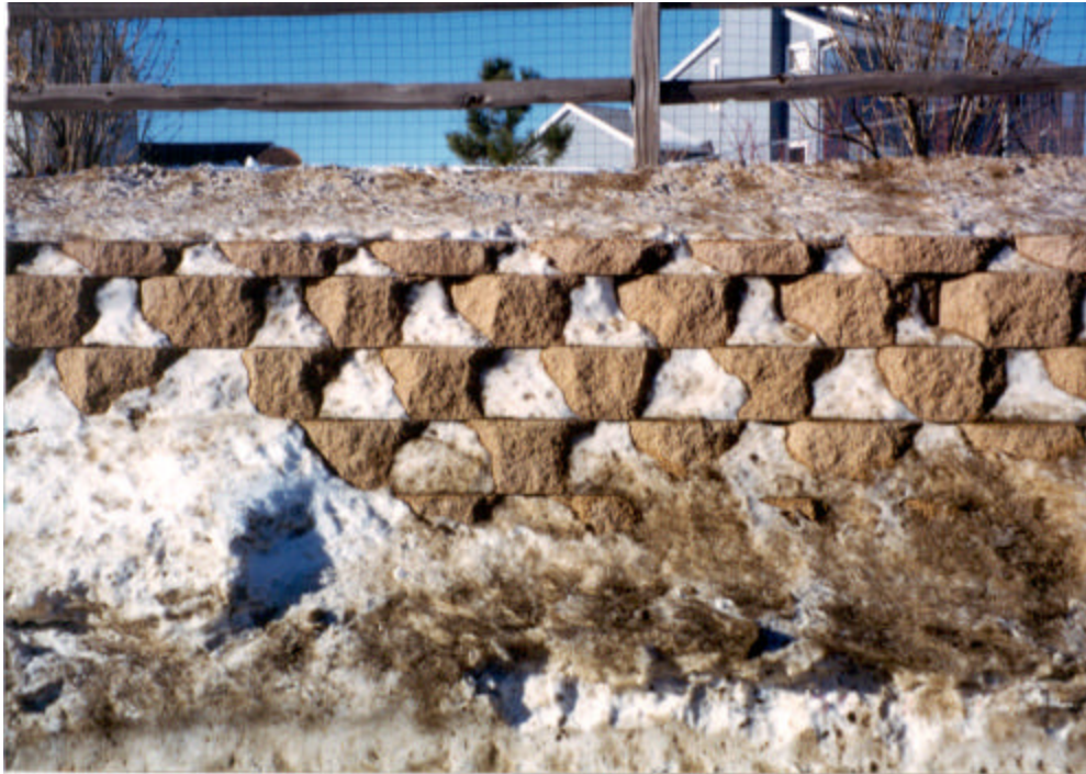
Figure 4.67. Photo illustrating the effect of fencing on snow accumulation (CSAH 101 and 87 th Place [west SCBRW]).
