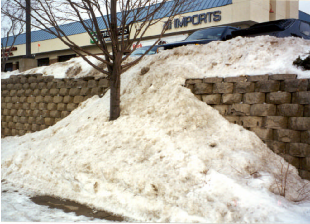
Figure 4.13. Close-up photo of snow accumulation from parking lot snow removal on SCBRW subjectively rated as “poor”.
