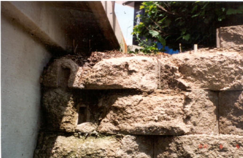
b. SCBRW located on east side of pedestrian bridge.
