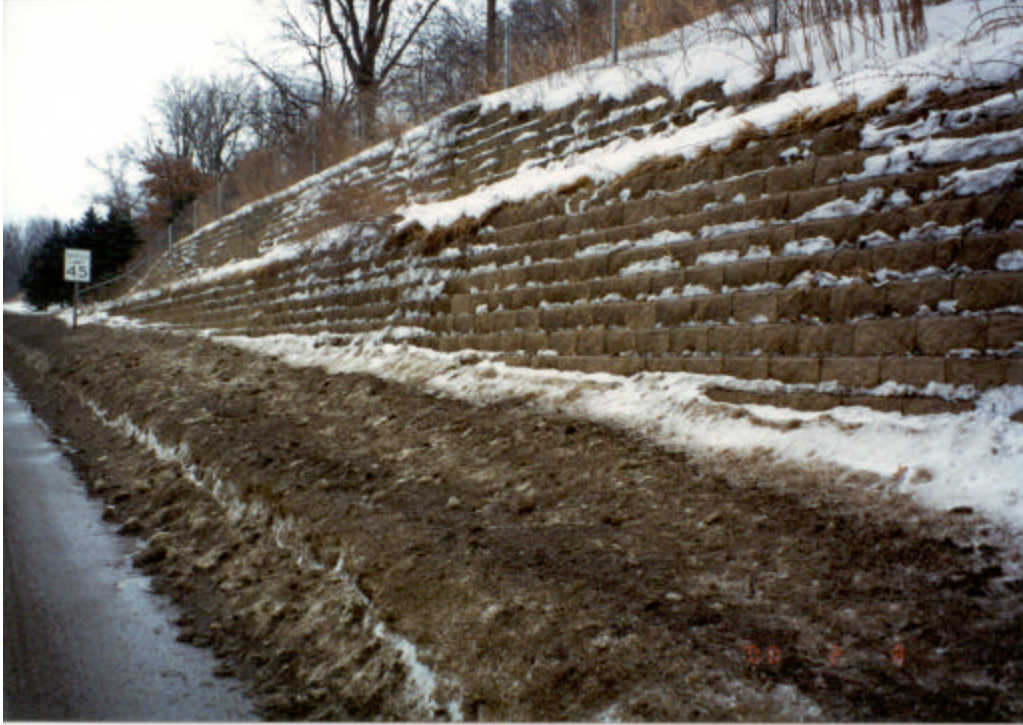
Figure 4.70. Photo illustrating high quantity of deicing sand/salt in snow accumulation (CSAH 38 and Gardenview).
