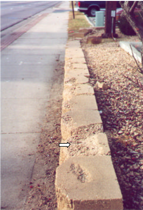
High-Severity Capstone Surface Scaling
