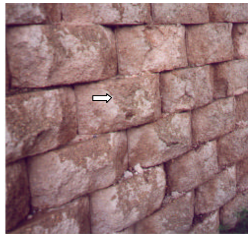
High-Severity Vertical Surface Scaling
