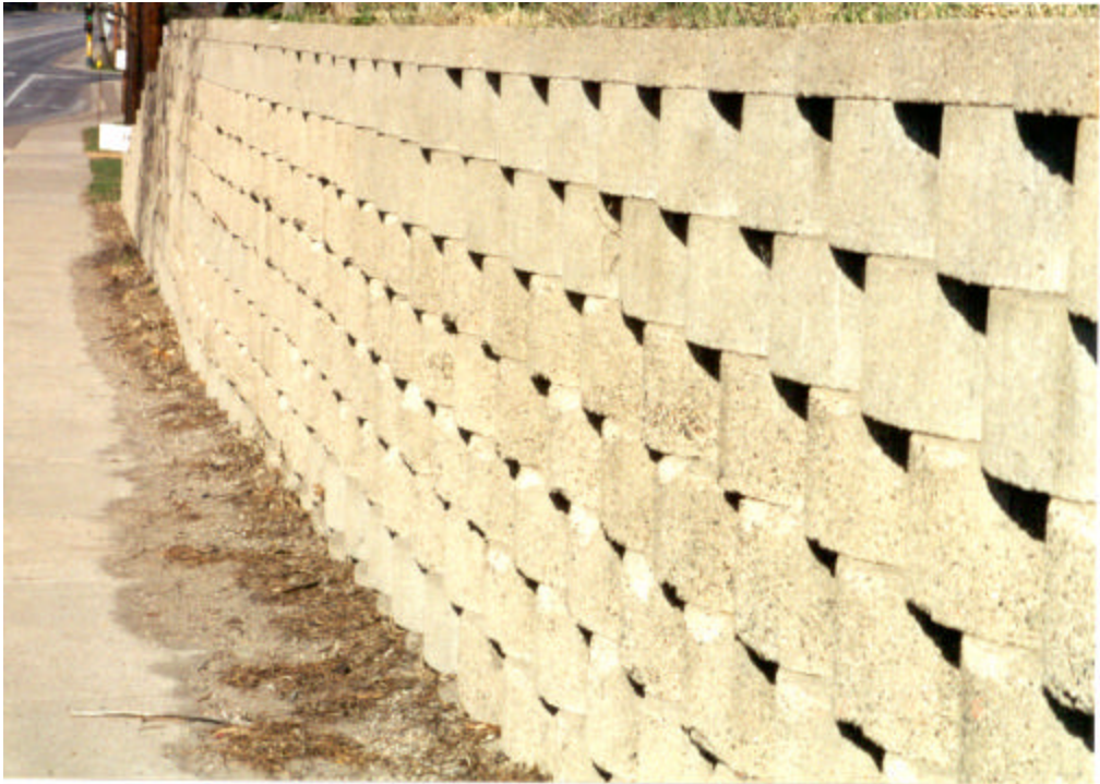
Figure 4.52. Example of apparent variations in mix design affecting block performance (CSAH 6 and 481 ft East of Dunkirk (north side)).
