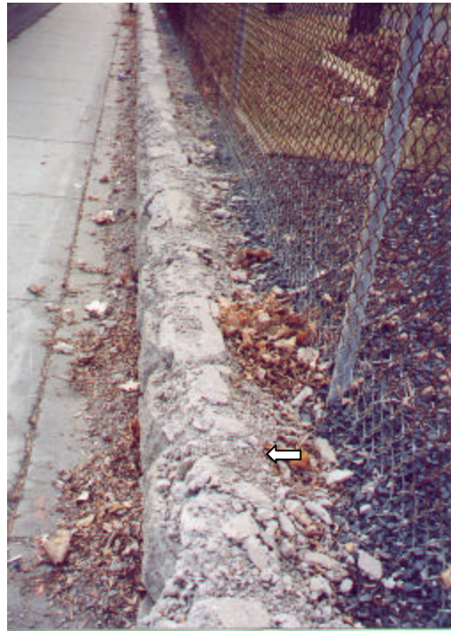
High-Severity Capstone Surface Scaling
