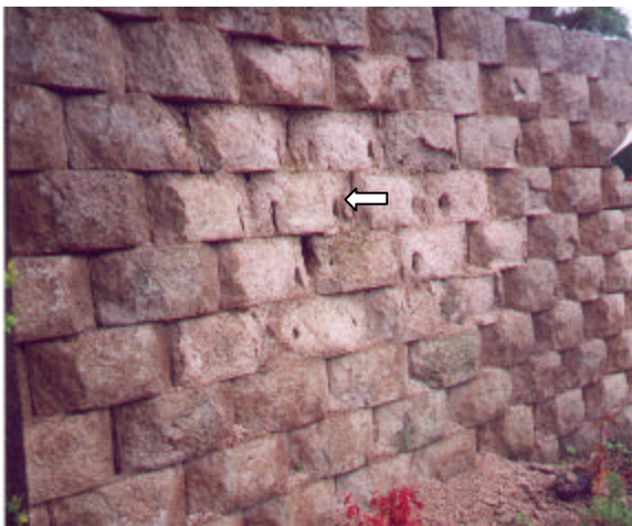
High-Severity Vertical Surface Scaling
