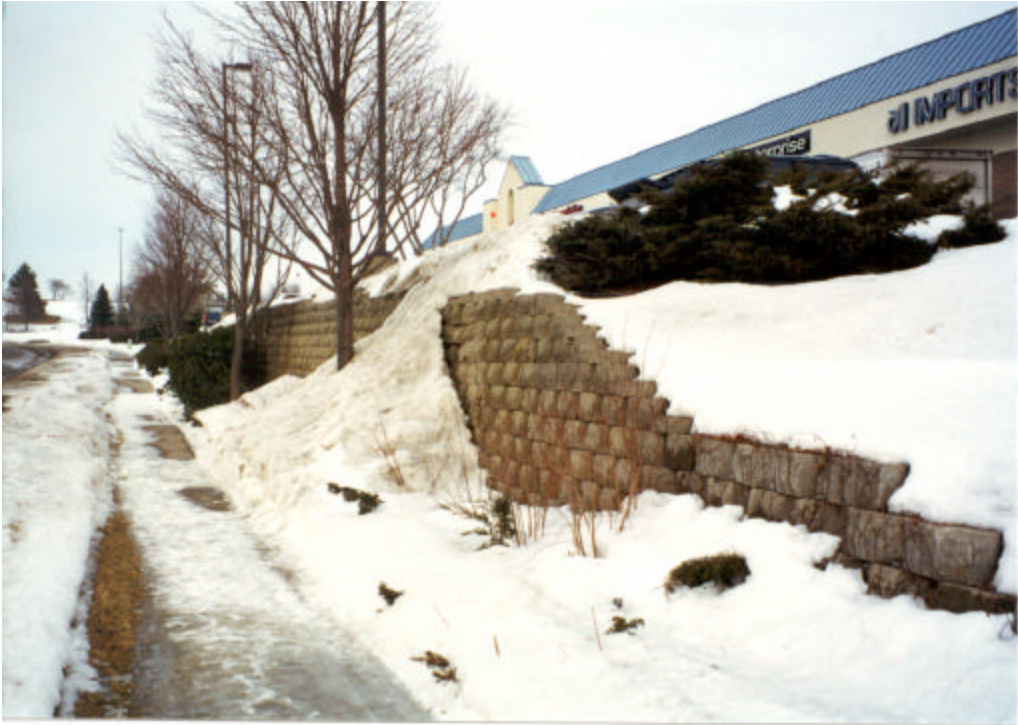
Figure 4.12. Overall photo of snow accumulation on SCBRW subjectively rated as “poor”.
