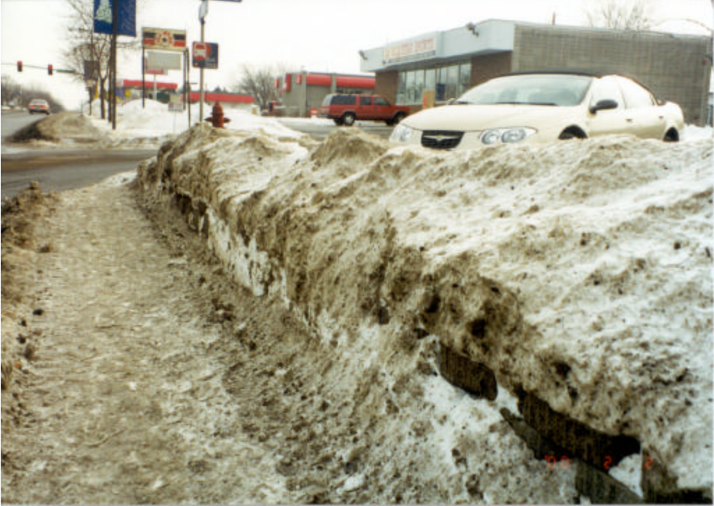
Figure 4.7. Photo of snow accumulation on SCBRW subjectively rated as “very poor”.
