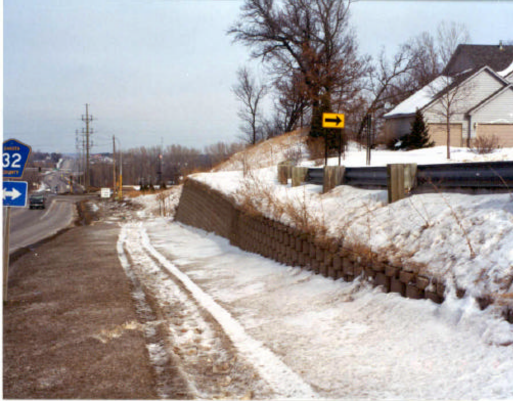
Figure 4.66. Photo illustrating the effect of the type of snow removal and offset distance on snow accumulation and quantity of deicing chemicals (SE Quadrant of Pilot Knob and Cliff Road).
