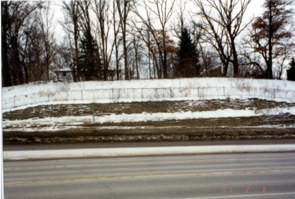
Figure 4.18. Overall photo of snow accumulation on SCBRW subjectively rated as “fair”.
