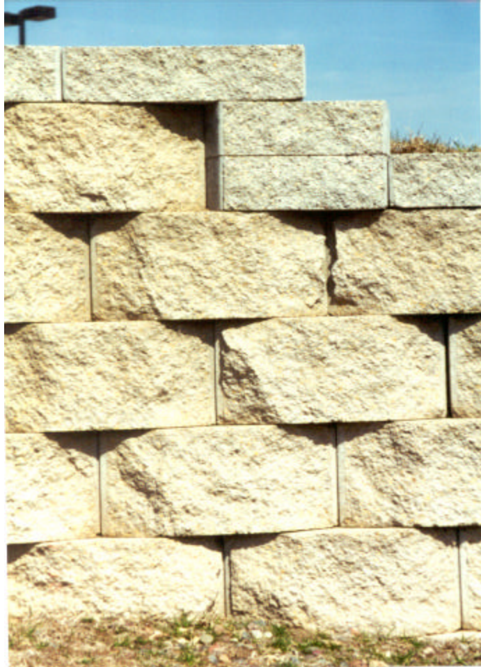
Figure 4.32. Close-up photo of general condition of masonry units used in SCBRW subjectively rated as “very good”.
