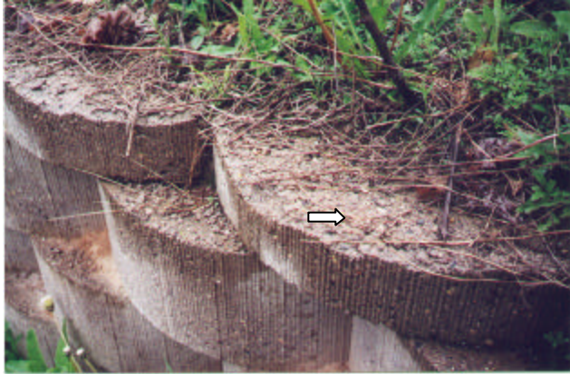
Medium-Severity Top Block Layer Scaling
