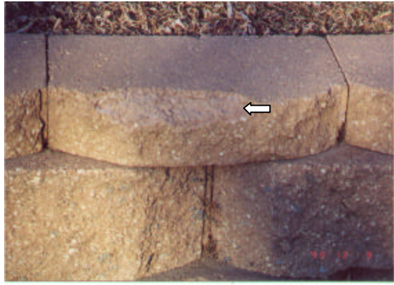
Medium-Severity Top Block Layer Scaling
