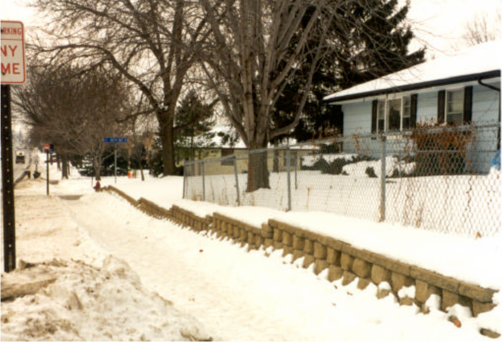
Figure 4.22. Overall photo of snow accumulation on southern SCBRW subjectively rated as “good”.
