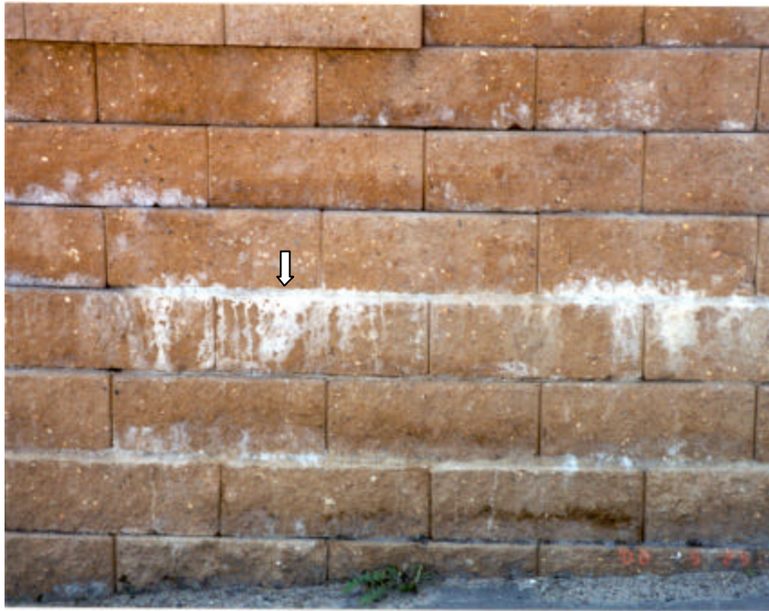
High-Severity Efflorescence
