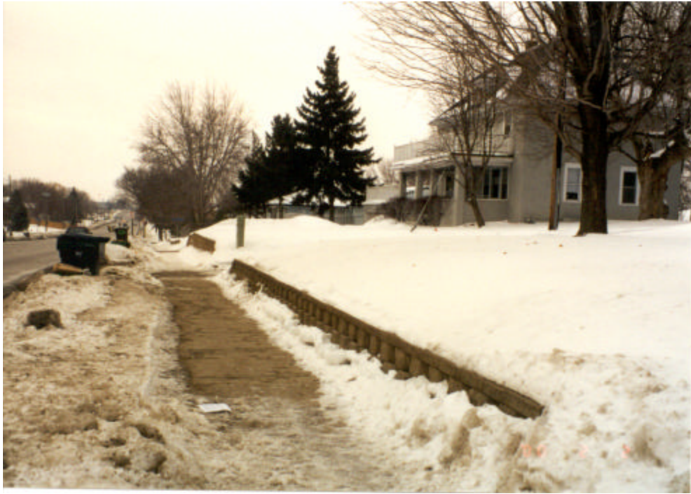
Figure 4.24. Overall photo of snow accumulation of northern SCBRWs subjectively rated as “good”.
