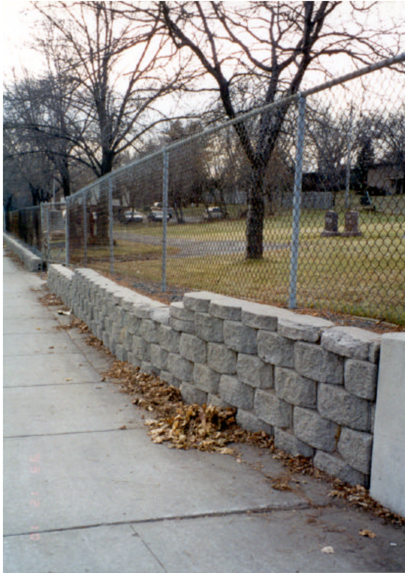
Figure 4.35. Photo illustrating reduced freeze-thaw deterioration at a location of minimal water runoff.
