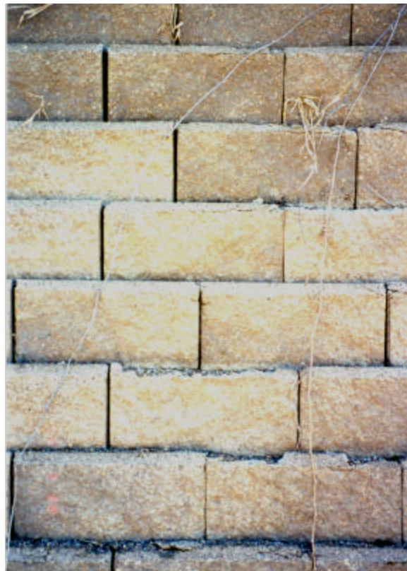
Figure 4.20. Close-up photo of high-severity position guide damage (high-severity freeze-thaw damage) on SCBRW subjectively rated as “fair”.
