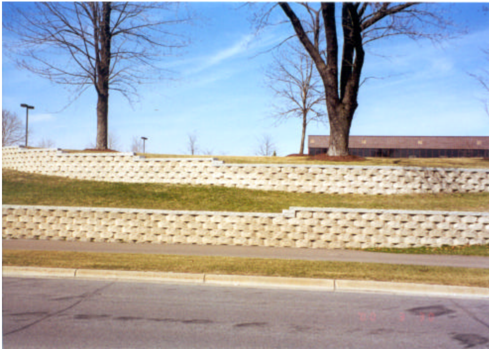
Figure 4.30. Overall condition photo of SCBRW subjectively rated as “very good”.
