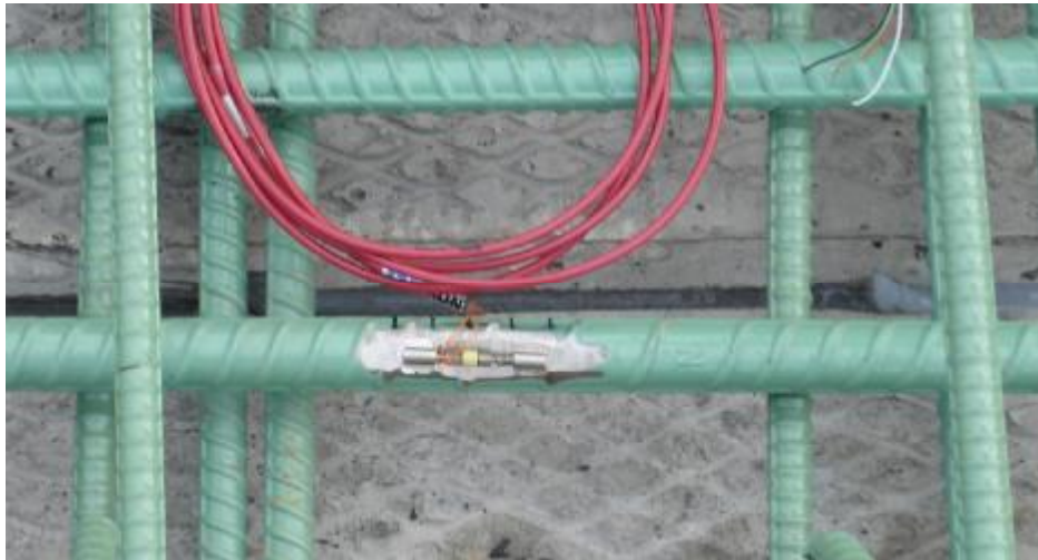
Figure 4.16 Photograph of VW spot-weldable strain gage welded to longitudinal reinforcement
