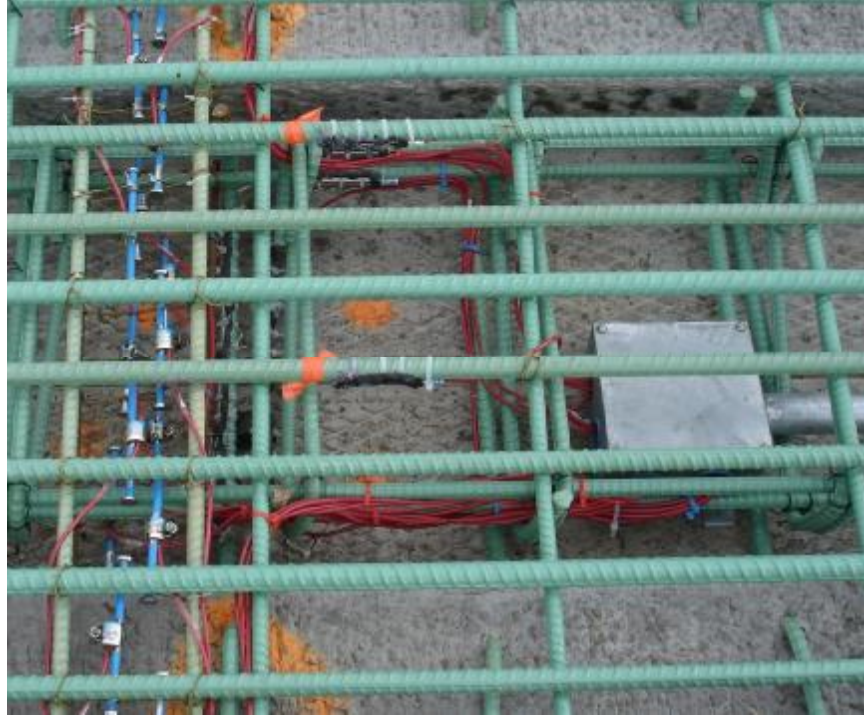
Figure 5.4 Photograph of embedded wiring junction box located above precast longitudinal joint
