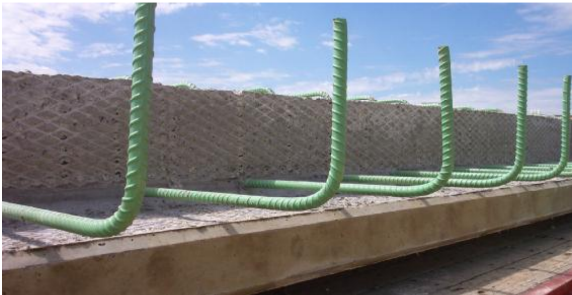
Figure 3.3 Photograph of the transverse hooks of the precast sections
