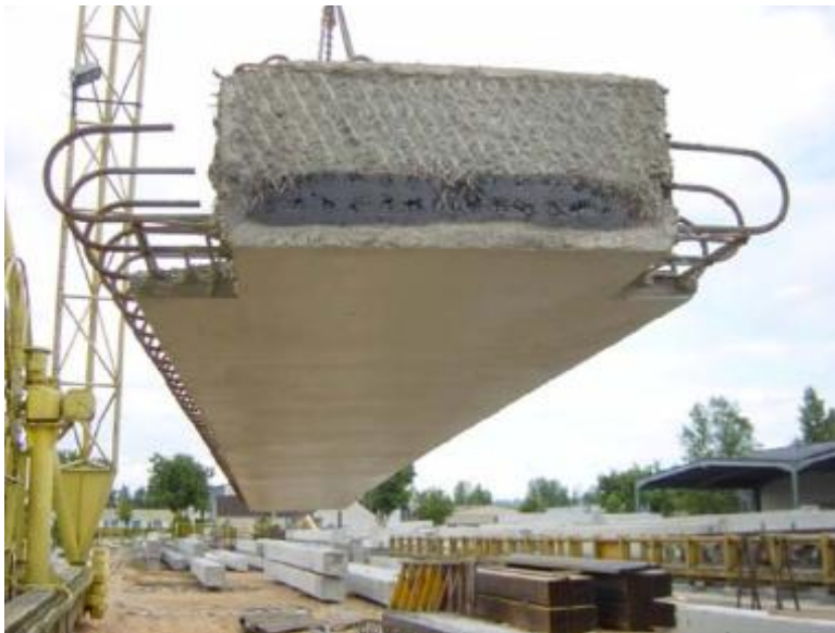
Figure 1.3 Photograph of precast section used in Poutre Dalle System (Hagen, 2005)
