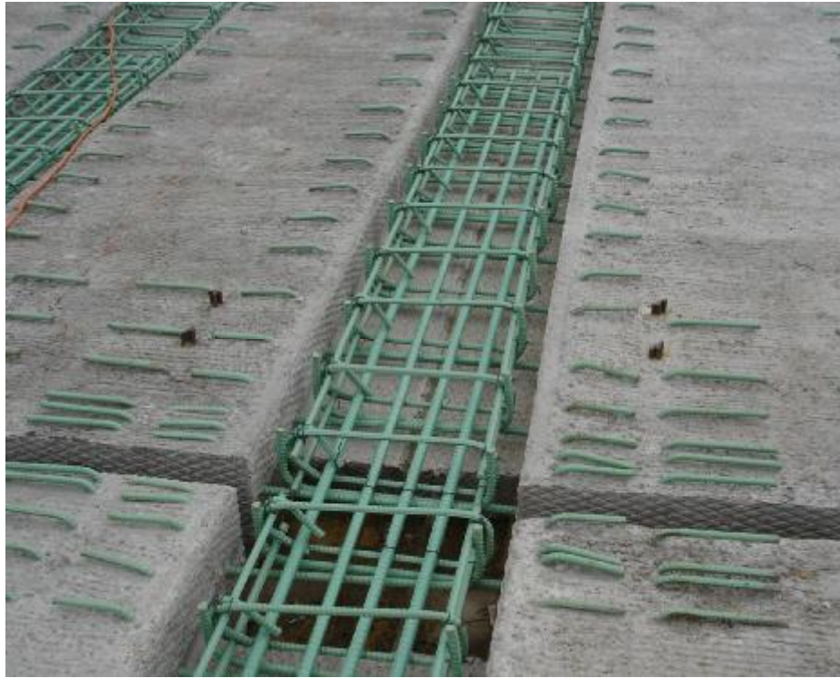
Figure 3.8 Photograph of the reinforcement cage installed above the precast longitudinal joint
