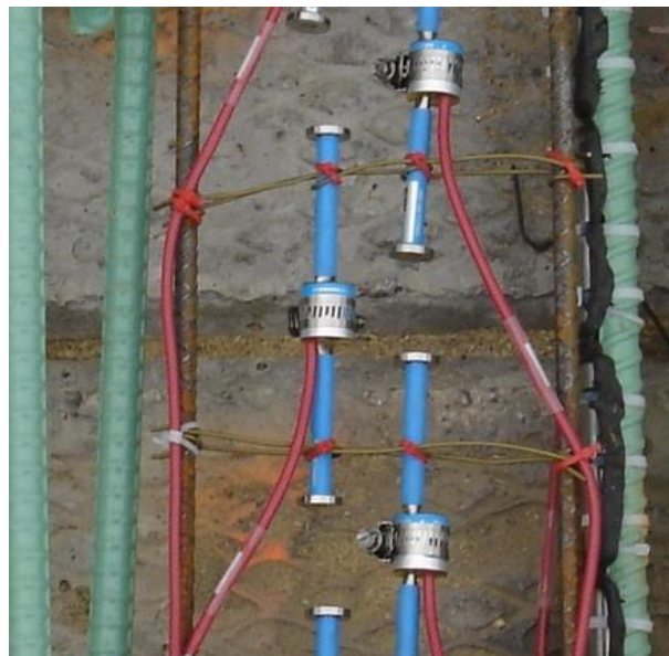
Figure 4.6 Photograph of VW embedment strain gage tied to uncoated rebar
