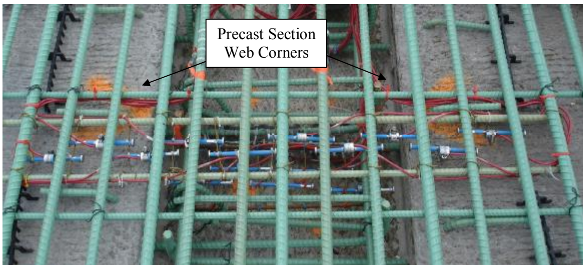
Figure 4.10 Photograph of VW embedment strain gages installed above precast section web corners and above precast longitudinal joint
