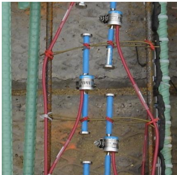
Figure C.2 Photograph of VCE-4200 VW Embedment Strain Gage tied to uncoated rebar
