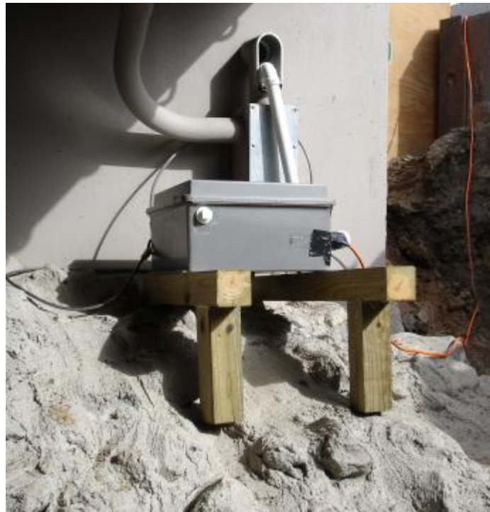
Figure 5.7 Photograph of temporary data acquisition system cabinet
