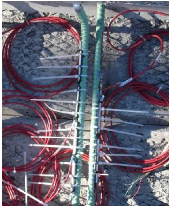
Figure 4.22 Photograph of VW spot-weldable strain gages on transverse hooks
