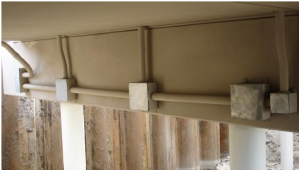
Figure 5.5 Photograph of multiplexer boxes located on the east face of the east pier cap (north is to the right)
