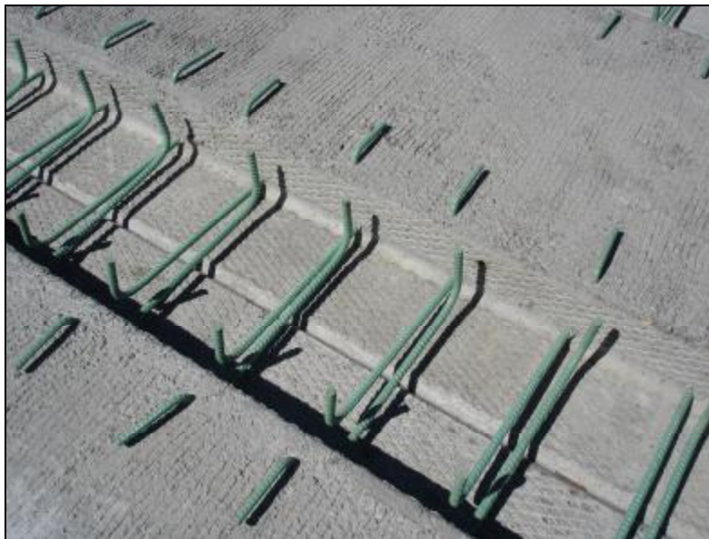
Figure 4.20 Photograph of transverse hooks of adjacent precast sections
