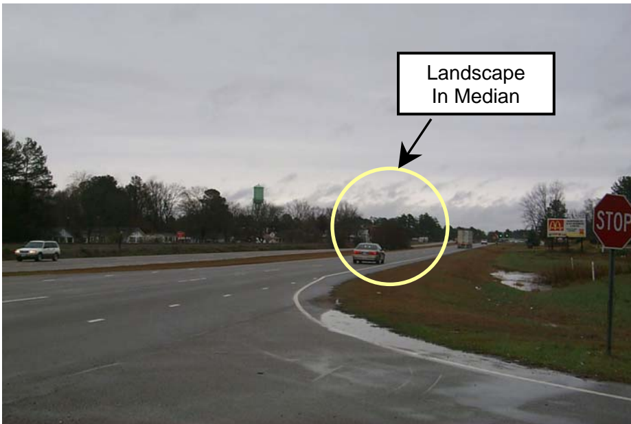
FIGURE 5-11 Median Landscaping Along US 74 (looking east from south approach)
