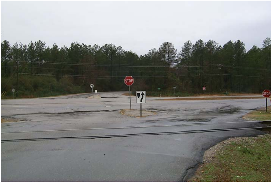
FIGURE 5-12 Location of Railroad Line (looking south at intersection)
