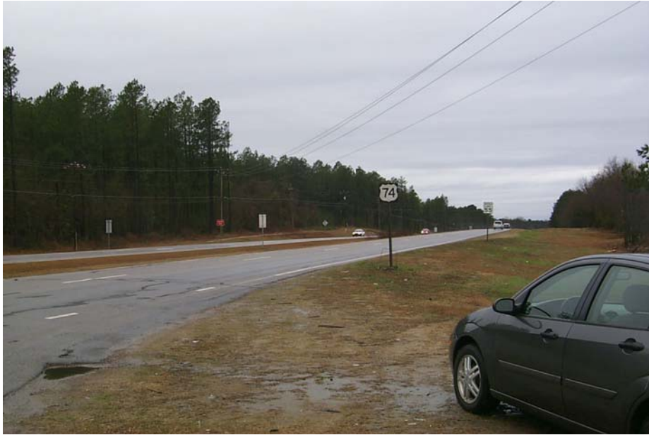
FIGURE 5-10 Grade Separation to the West of US 74 and SR 1152 Intersection (looking west from north approach)
