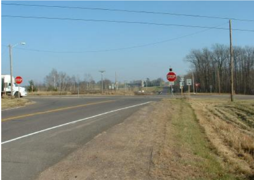
FIGURE 5-2 General Area at CTH V Intersection (west approach)
