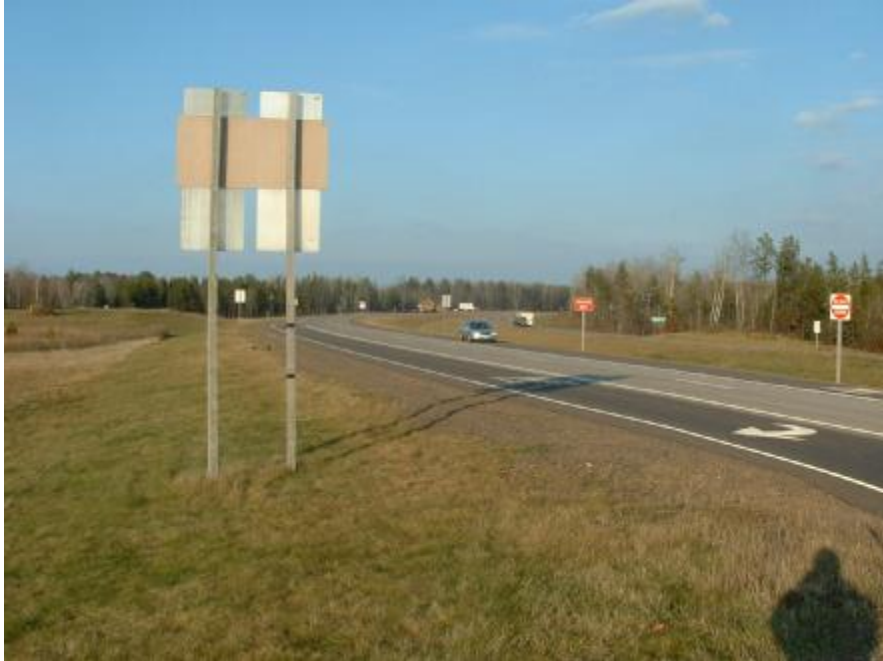
FIGURE 5-7 Horizontal Curve at STH 77 (looking north from west approach)
