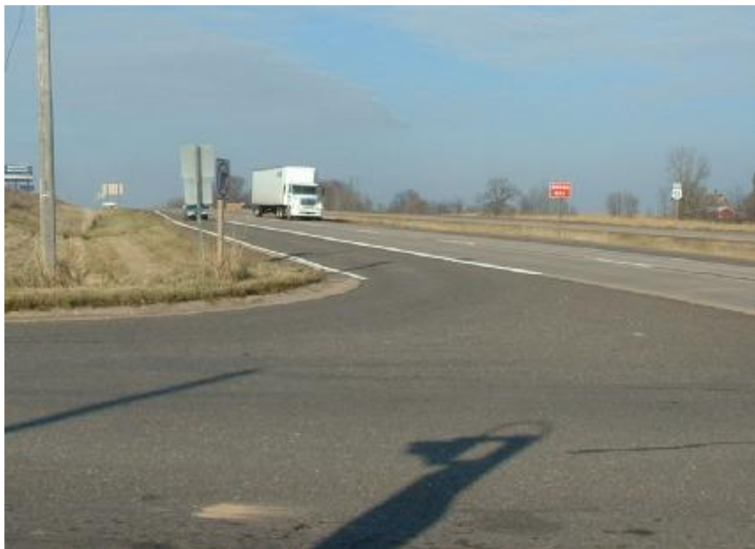
FIGURE 5-3 Crest Vertical Curve to North of CTH V Intersection (looking north from west approach)
