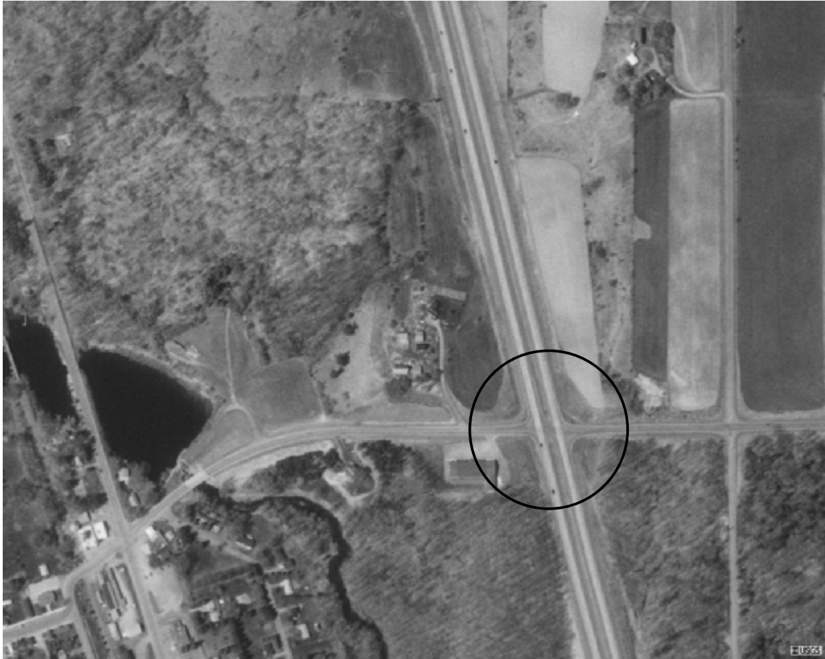
FIGURE B-1 Aerial Photo of U.S. 53 and CTH V (Barron County) Source: www.terraserver.com
