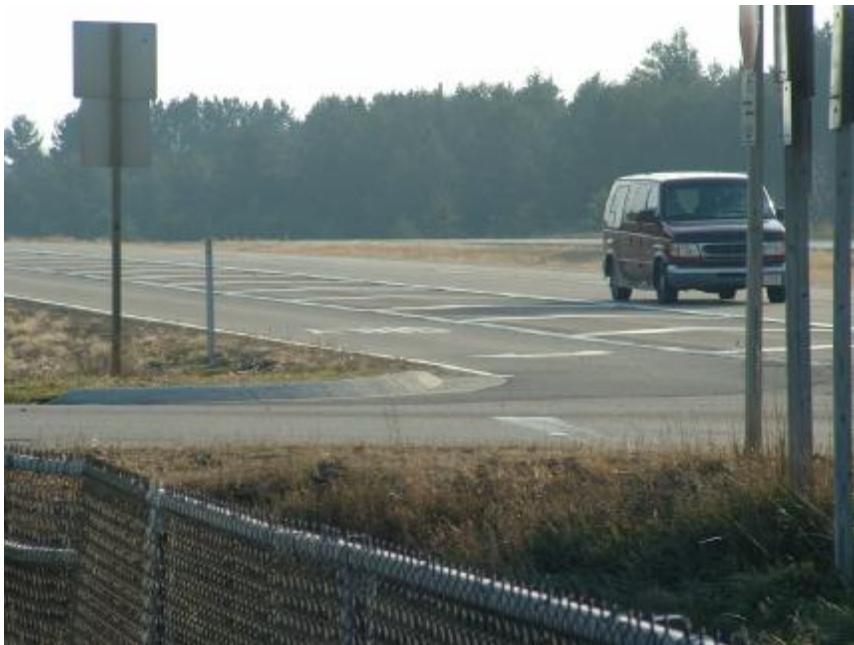
FIGURE 5-6 Example Offset Right Turn Lane at CTH E and U.S. 63 (looking south from east approach)
