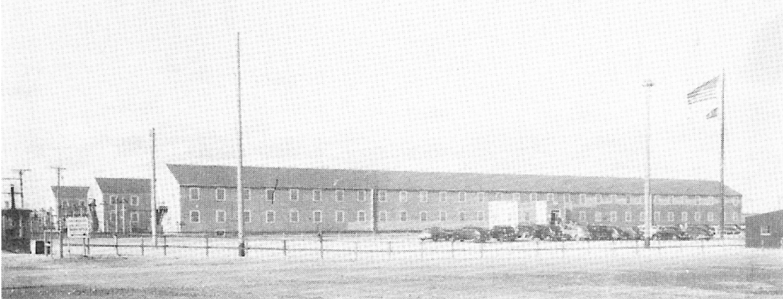
Figure 7. Building 703A was pressed into service as a polio hospital following the University's acquisition of the Rosemount property. It later housed geriatric patients from the Hastings State Hospital. The structure was demolished in 1978 to make way for an expansion of the Dakota County Vocational Technical Institute. U.S. Army Corps of Engineers.
