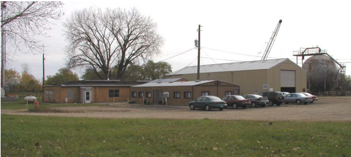
Figure 4. The same area as it appears today. The Ammonia Oxidation Building (302-A) containing the Rosemount Aeronautical Laboratory's wind tunnel equipment burned in 1976 and was replaced with a steel pole structure. The Morton Sphere is visible at right.
