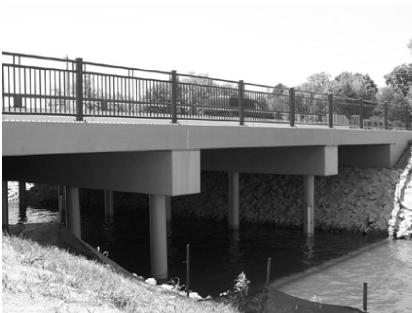
Figure 3.1: Photograph of the Center City Bridge
