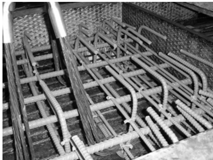
Figure 5.25: Rebar congestion at end of Center City Bridge precast section
