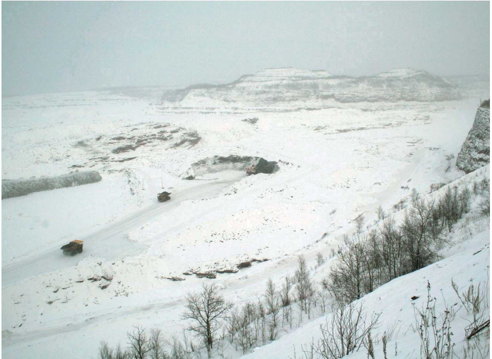
Fig. 3.24: Winter View from Existing "Mineview" Overlook. Hibbing, 2008.
