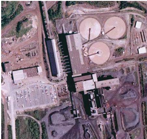
Fig. 4.10: Pellet Plant at Keetac. Year Built - 1967. Location - Keewatin, MN.
