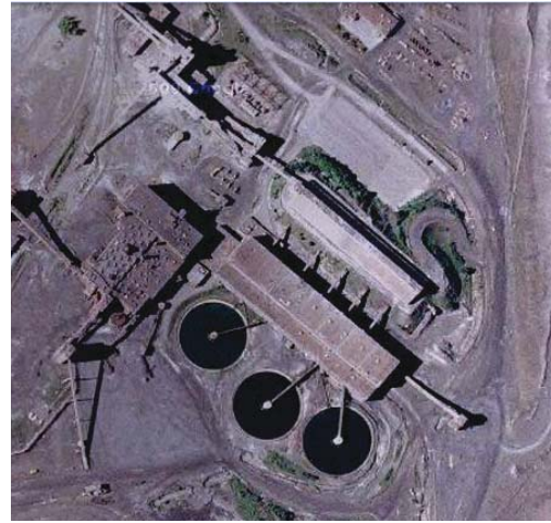
Fig. 4.8: Pellet Plant at United Taconite. Year Built - 1965. Location - Forbes, MN.
