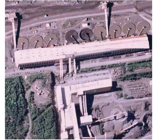
Fig. 4.9: Pellet Plant at Minntac. Year Built - 1967. Location - Mt. Iron, MN.
