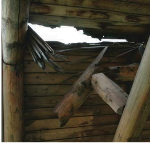
Fig. 6.2: Blast Damage near Hull-Rust Overlook.
