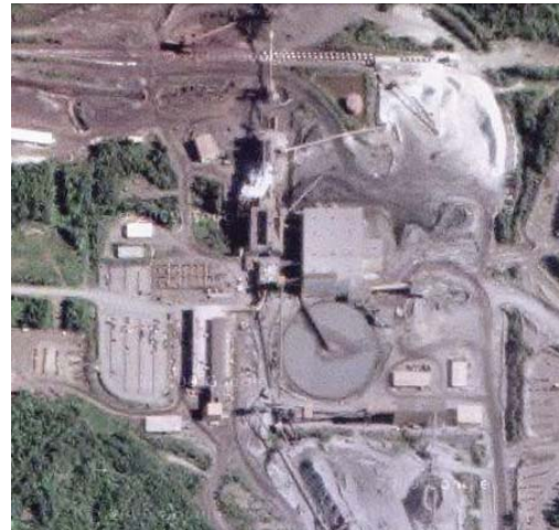
Fig. 4.11: Pellet Plant at the Minorca Mine. Year Built - 1974. Location - Virginia, MN.
