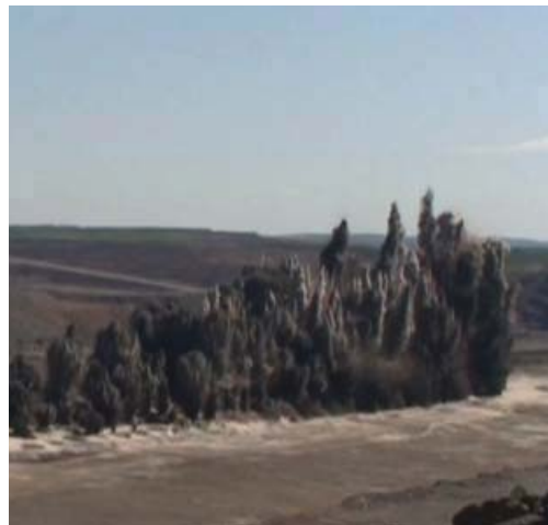
Fig. 4.16: Typical Mesabi Range Mine Blast.
