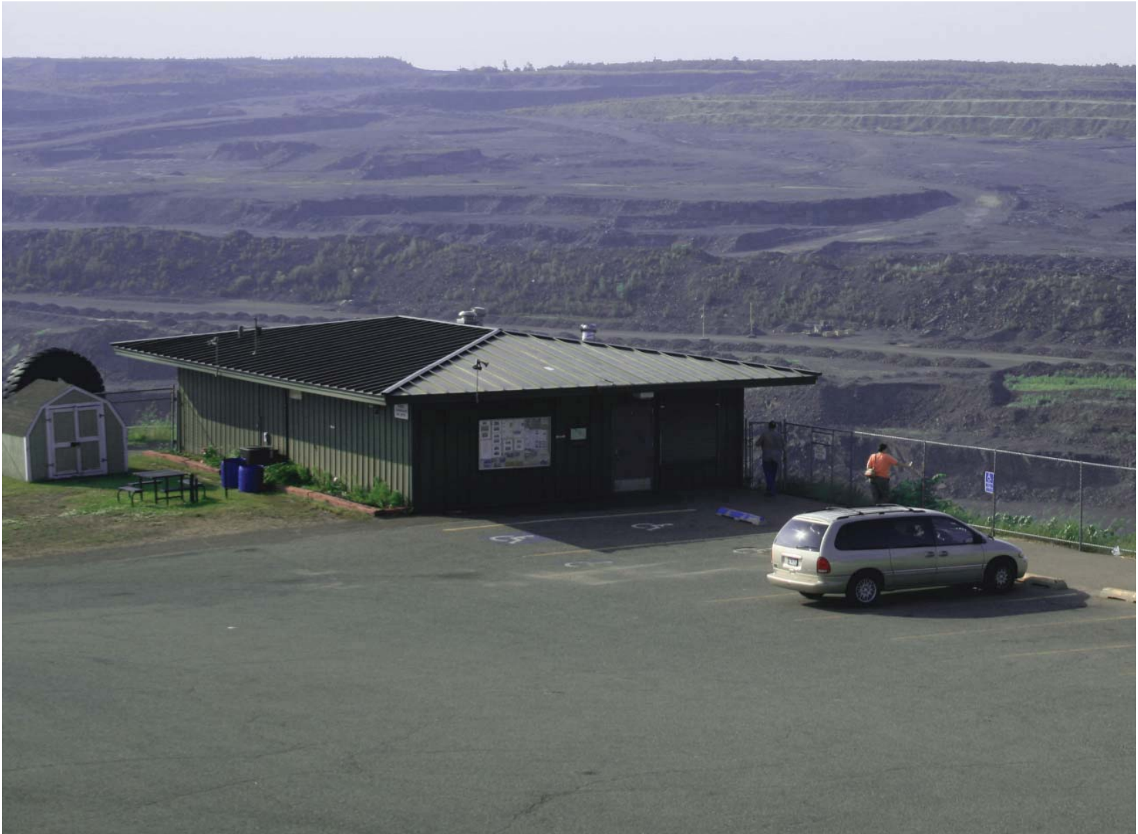
Fig. 3.25: Existing "Mineview" Overlook Structure. Hibbing, 2008.
