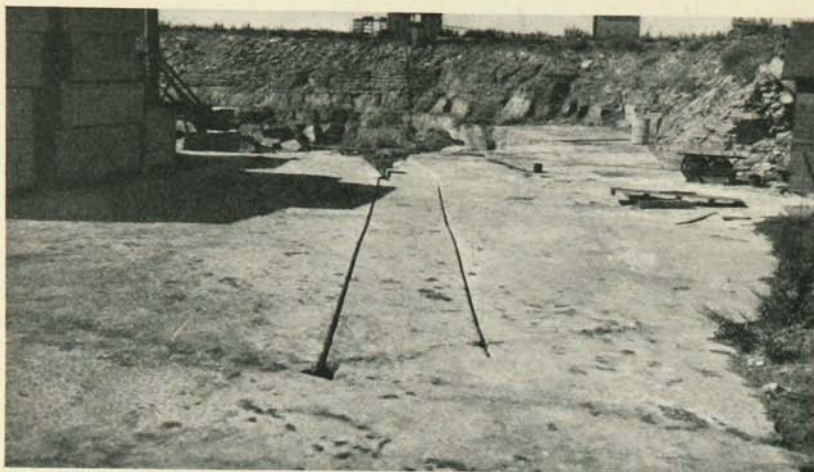
FIGURE 63.—A key block cut by a "channeler" in a ledge of the quarry of the Babcock and Wilcox Company near Kasota.
