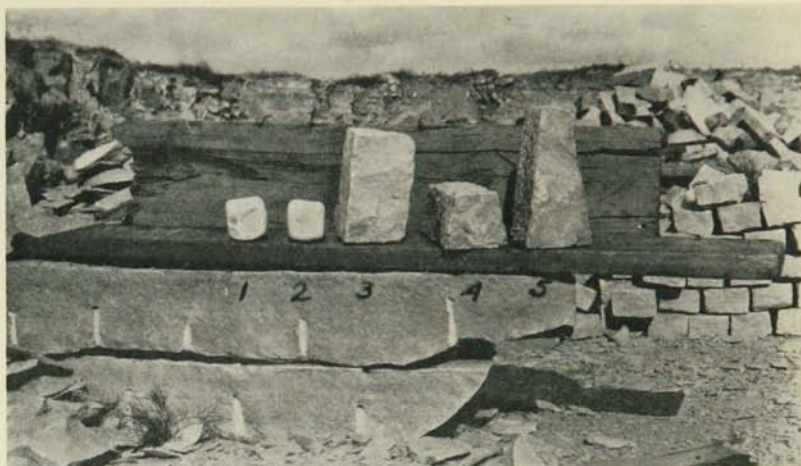
FIGURE 78.—Stone products made by Jasper Stone Company. 1. Eight-hour grinding pebble. 2. Eleven-hour grinding pebble. 3. Regular lining block. 4. Wedge-shaped lining block for side of mill. 5. Wedge-shaped lining block for end of mill.
