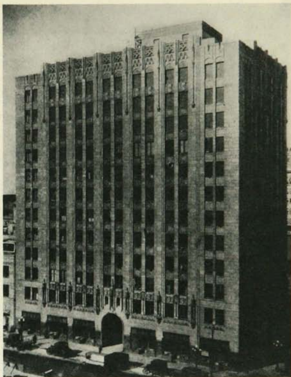
FIGURE 76.—The Baker Building in Minneapolis. The base course is Morton granite and the upper exterior is Kettle River sandstone.
