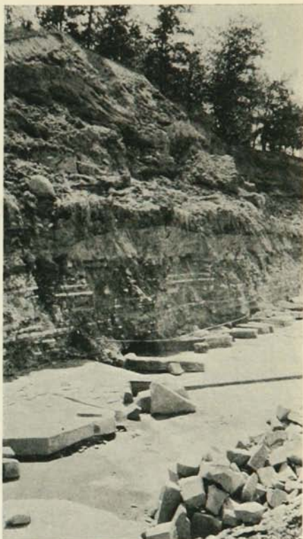
FIGURE 74.—Lieb's Quarry at Faribault. An overburden 60 feet thick of glacial drift and decomposed dolomite covers the ledges.
