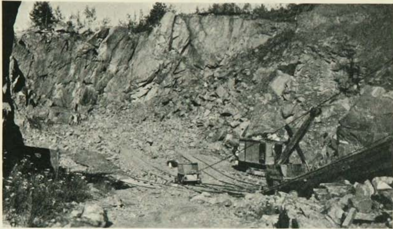
FIGURE 59.—Quarry of the B. F. Nelson Company in Archean greenstone near Ely. The rock is crushed and screened for roofing granules.
