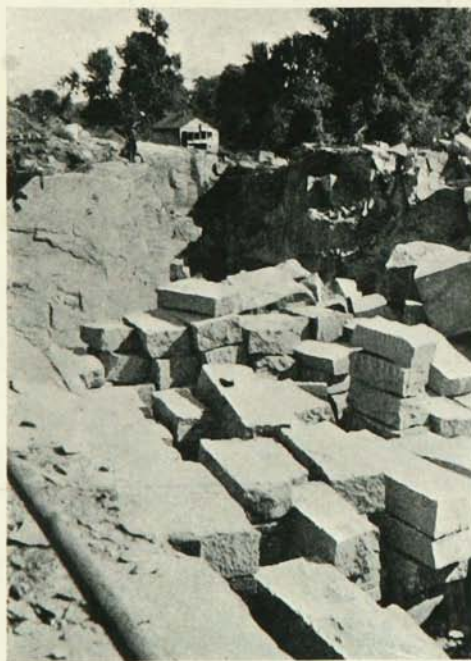
FIGURE 51.—The quarry of the Rock Valley Granite Company south of the village of Sacred Heart in Renville County.
