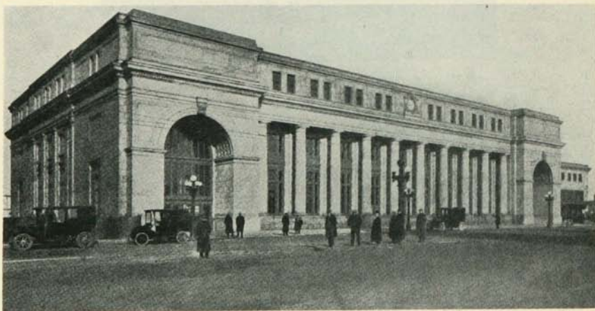
FIGURE 77. — The Great Northern Union Depot, Minneapolis. Constructed of sandstone from the Kettle River quarries. Photograph by Bowles.
