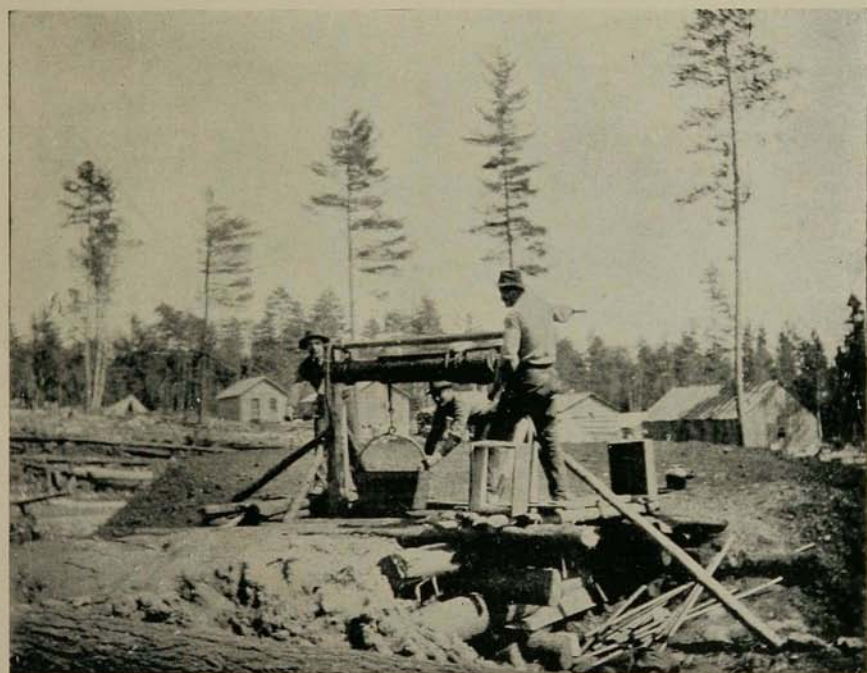
TEST-PITTING AT THE BIWABIK MINE.
