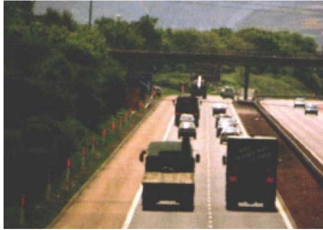
Figure B-8. COMPANION roadside warning lights, which cover a 4 km section of highway in Scotland.
