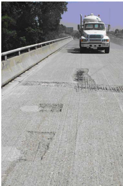
Figure 4.1 Milled deck, and Type 1 Repairs before Reoverlaying
