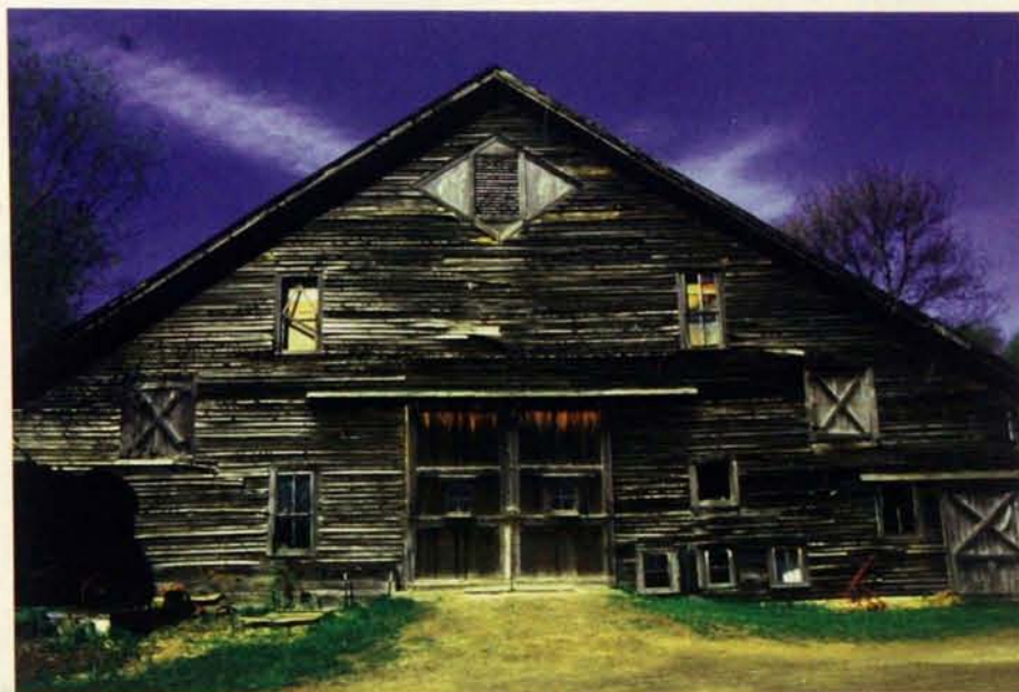
A NORTHERN PACIFIC RAILROAD BARN, CIRCA 1875, LOCATED ON THE STAGECOACH ROAD NORTH OF ANOKA. THE BARN WAS USED AS AN OVERNIGHT SHELTER FOR TRAVELERS ON THE STAGE LINE.
