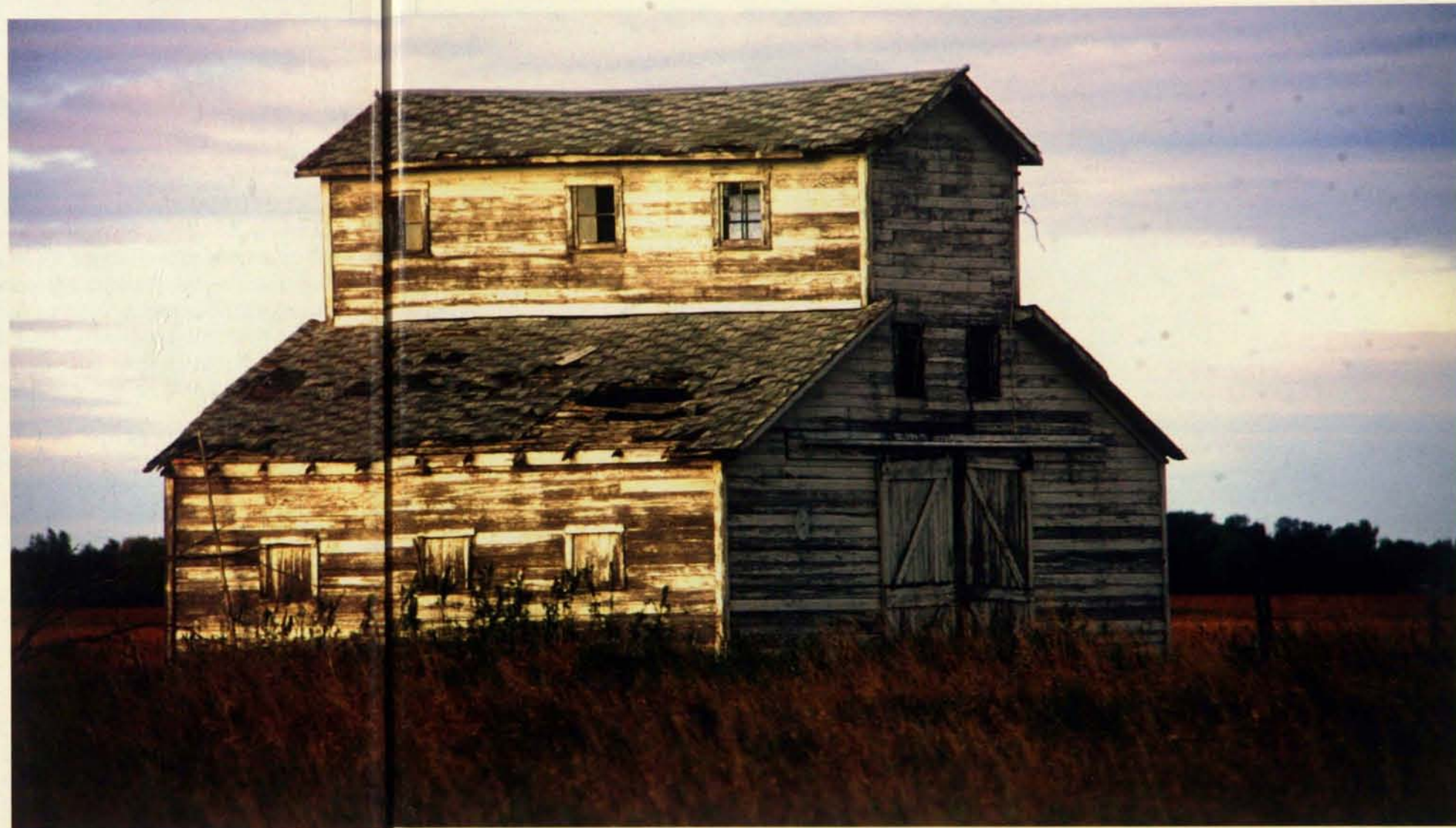
A MONITOR-ROOF HAY BARN, CIRCA 1925, IS ALL THAT REMAINS OF A RED RIVER FARM IN POLK COUNTY.
