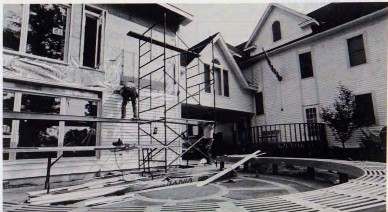
The addition on the Ronald McDonald House at 621 Oak Street SE is nearly complete.
