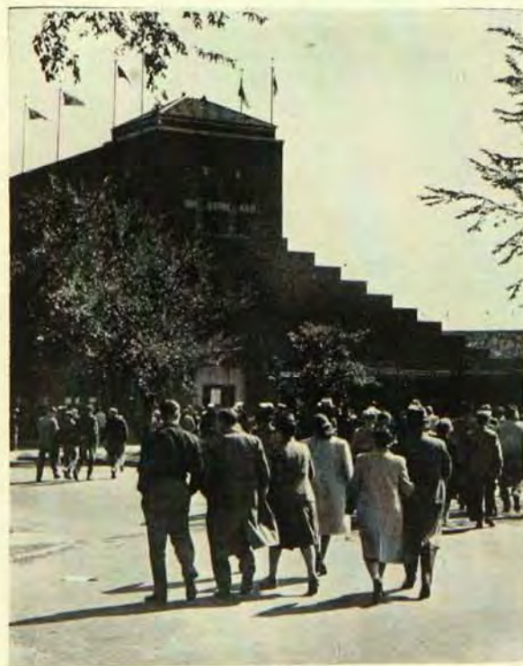
North Tower, Memorial Stadium
