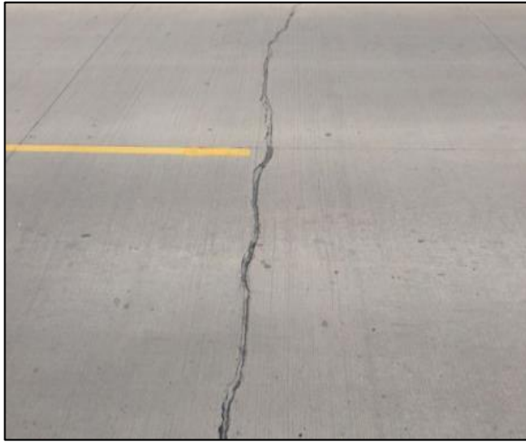
Figure 2.1: Transverse crack (left) and Longitudinal crack (right) (Harrington et al., 2018).
