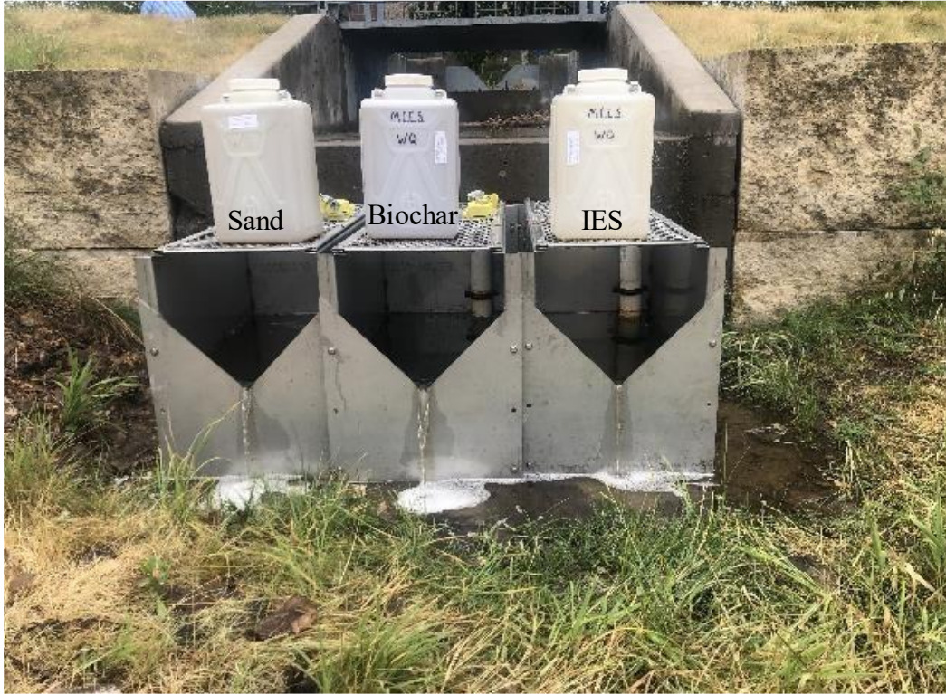
Figure 3. Effluent Weir Boxes for Filter Testbeds
