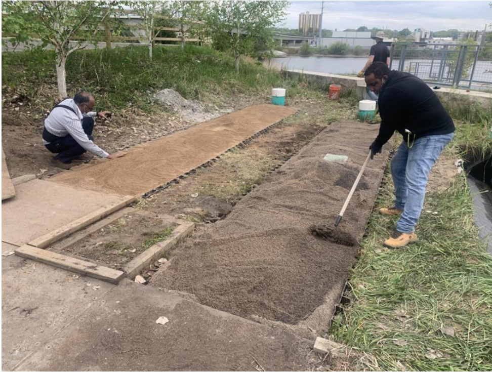
Figure 5. Raking the Biochar Filter
