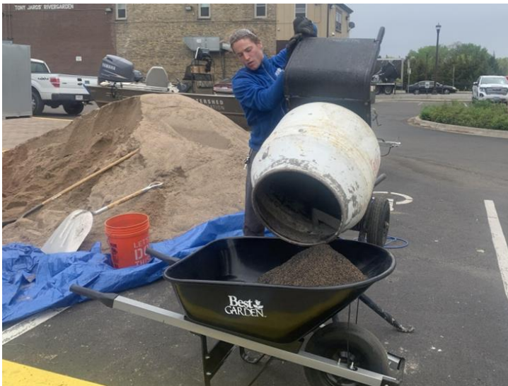
Figure 4. Using a Cement Mixer for Biochar and Sand Mixing
