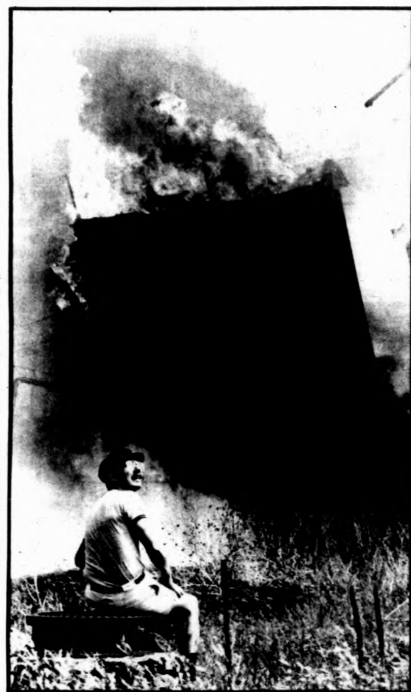
One interested onlooker, sitting on a manhole cover east of the burning grain elevator, watched the spectacular fire and hovering television helicopters.
