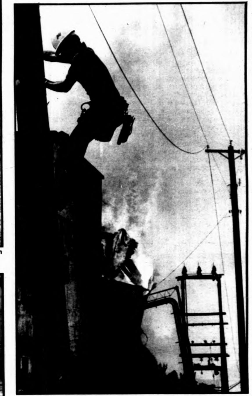
Northern States Power lineman Steve Anderson climbed down from a utility pole after he disconnected one of the power lines close to the fire. One of the building's walls collapsed shortly afterwards.
