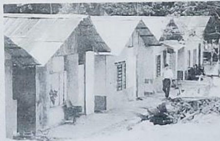
ILLEGAL CLUSTER: The units near Pinggiran Ukay
