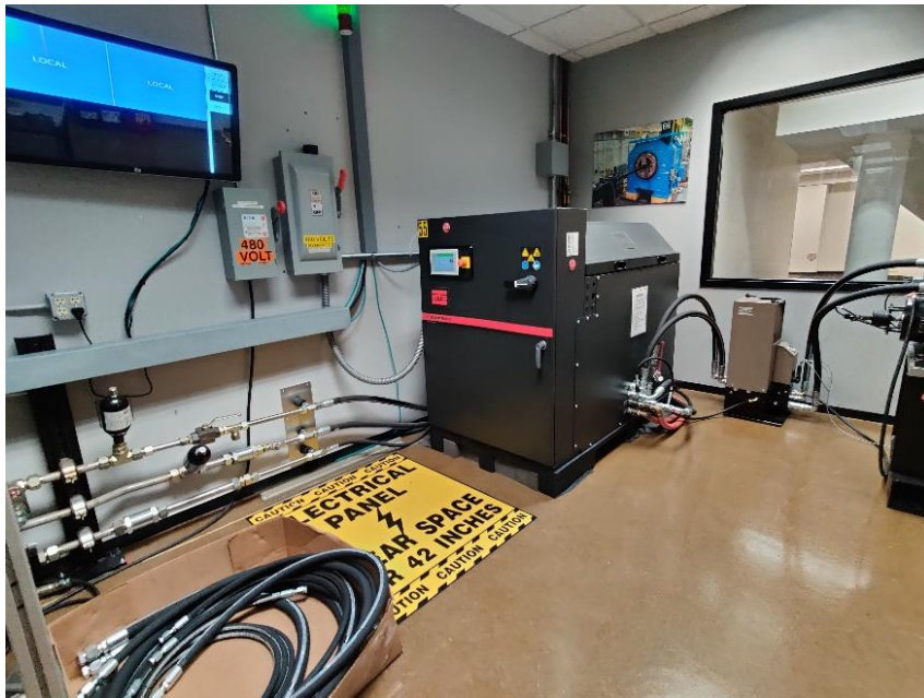
Figure 2.5 Hydraulic Power Unit : The pump unit in the corner of the test lab that powers the loadframes in Figure 2.4
