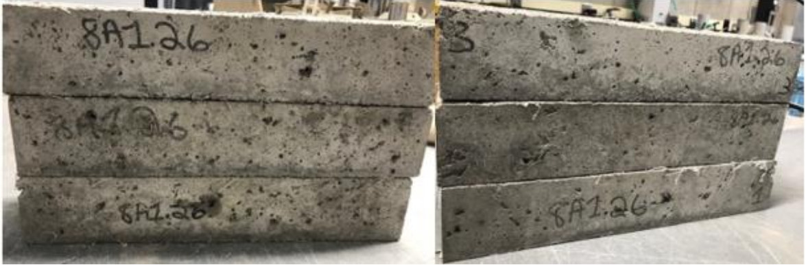
Figure 0-34. Image of mix 8A1.26 beams after 300 freeze-thaw cycles
