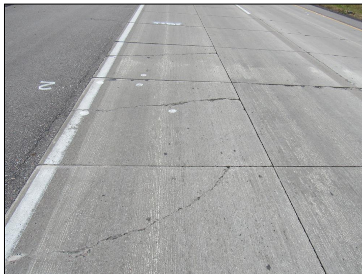
Figure 3-9: Transverse and Diagonal Cracks Observed in Cell 506 (October, 2019).
