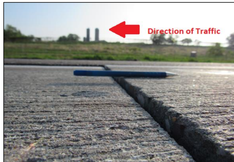
Figure 3-7: Faulting in Cell 506 (no fibers).
