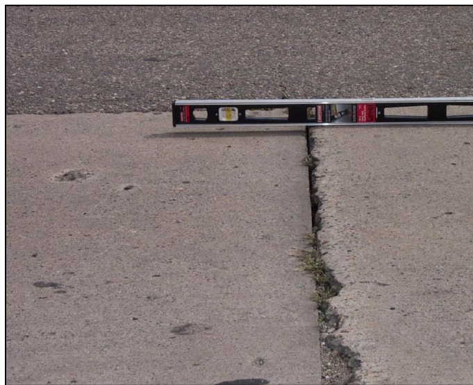
Figure 2-2: Transverse joint faulting in concrete pavements (MnDOT, 2011).
