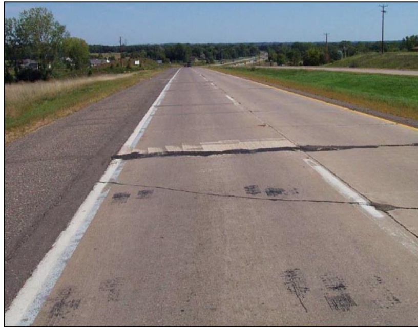
Figure 2-4: Concrete Pavement Slab Cracking (MnDOT, 2011).
