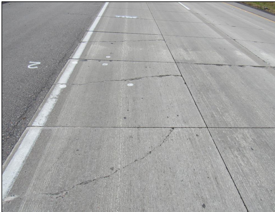
Figure 5-11: Cracks observed in Cell 506 (replaced in the summer of 2020).
