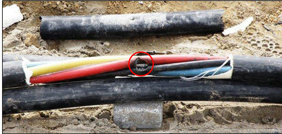
Figure 4. Failed underground electric cable [11].
