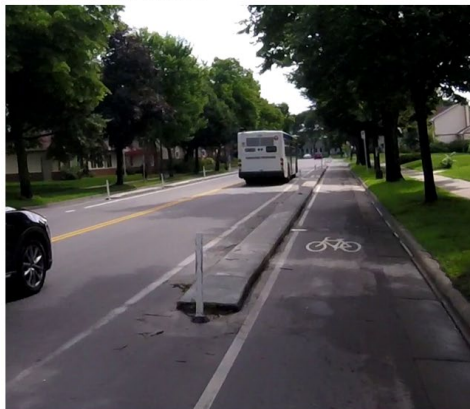
Buffer 3: Curb and Intermittent Barrier
