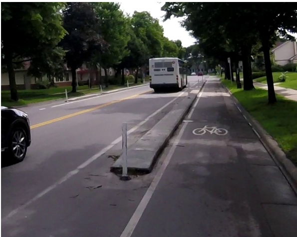
Buffer 3: Curb and Intermittent Barrier
