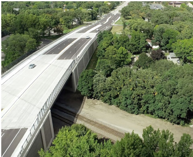
Hanson Boulevard railway grade separation
