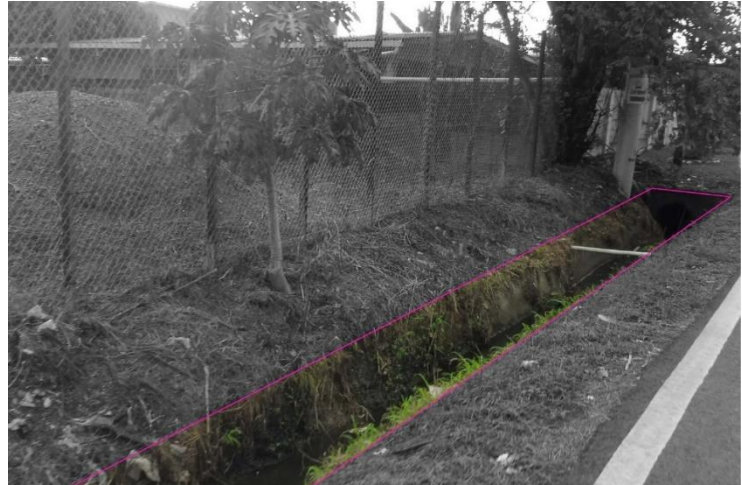
Figure 14 Makeshift Drainage Channels in Radial City Juan Diaz
