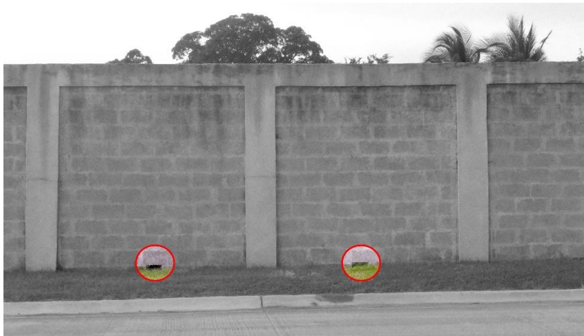
Figure 16 Wall Openings for drainage
